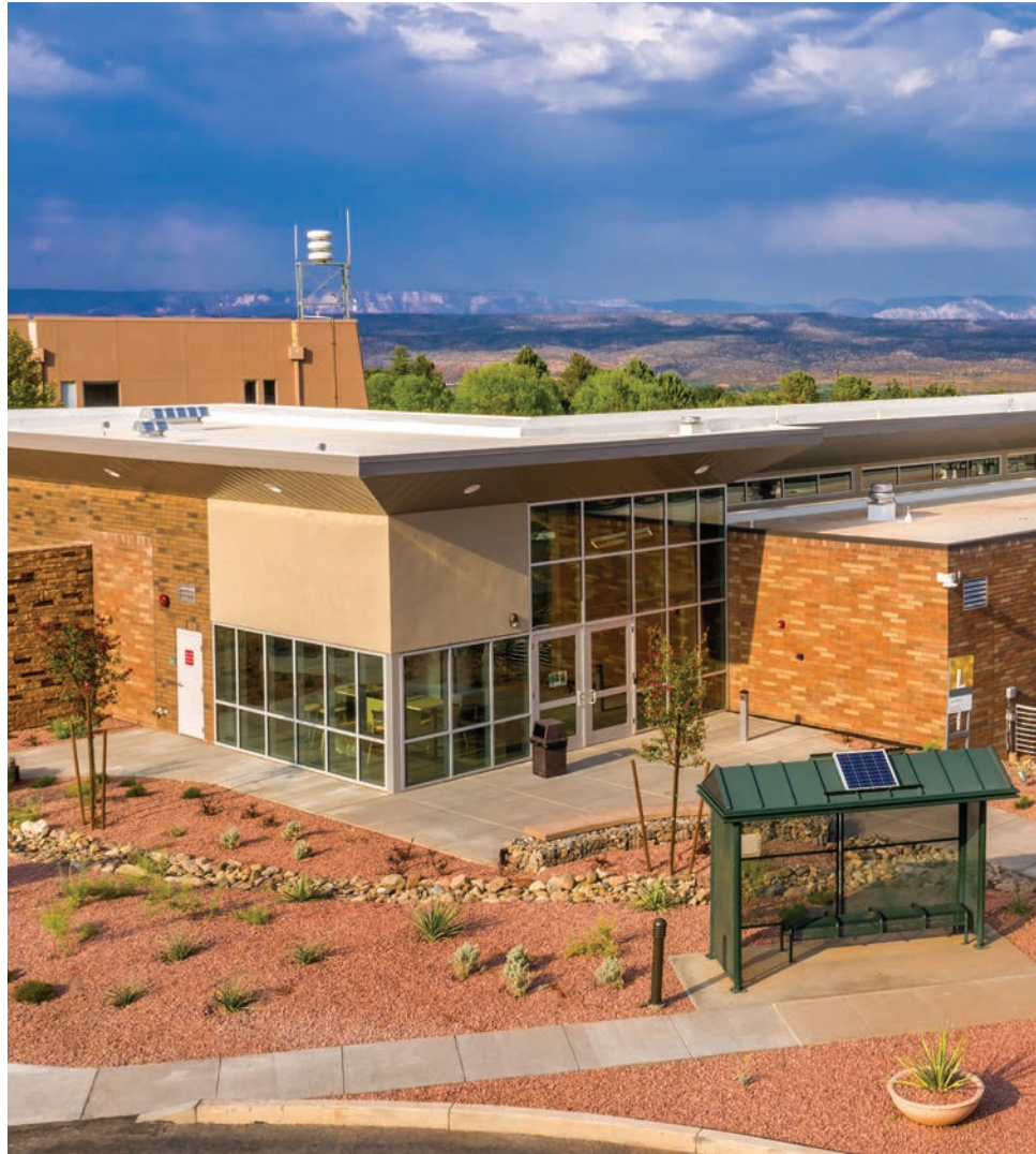
New front entrance of Building L
