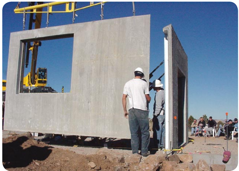
The Longview House features insulated, pre-fabricated concrete walls for the exterior basement.
