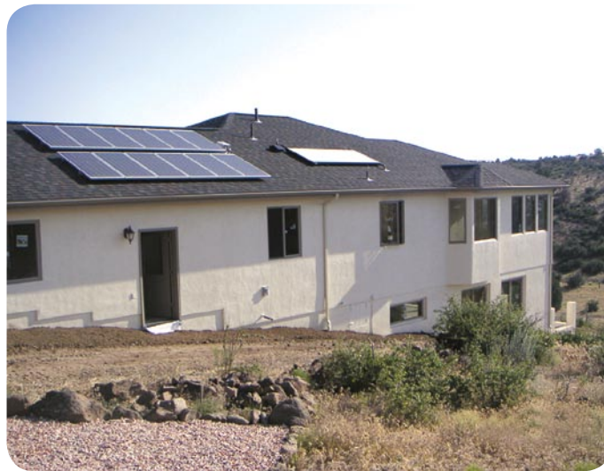
Active solar systems on the Longview House include a 2kW PV system and 4 ft. x 10 ft. solar collector for hot water. Note that the roof overhang shades with windows in this photo taken on the summer solstice.
