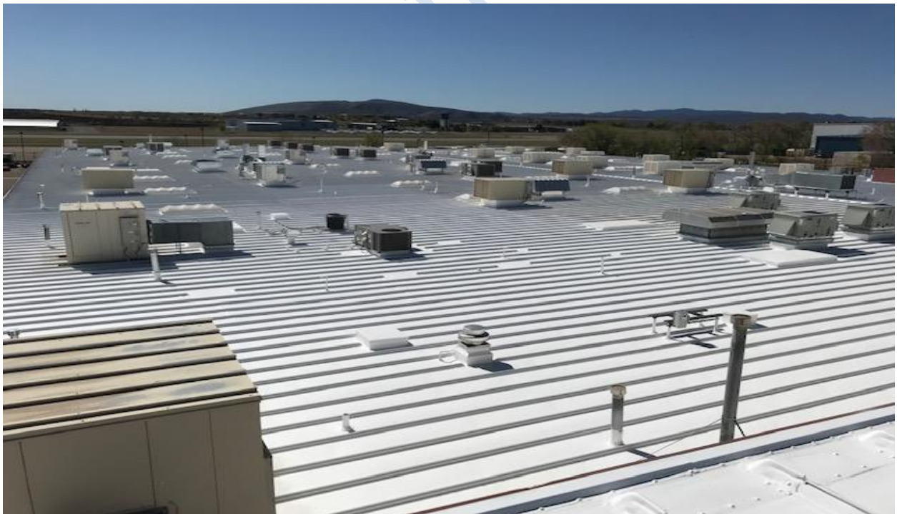
New Roof Coating at CTEC
