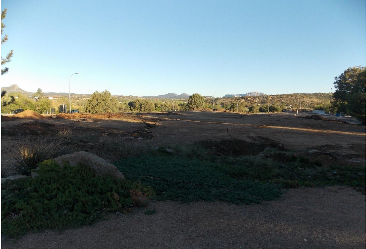
Site Leveling of New Field
