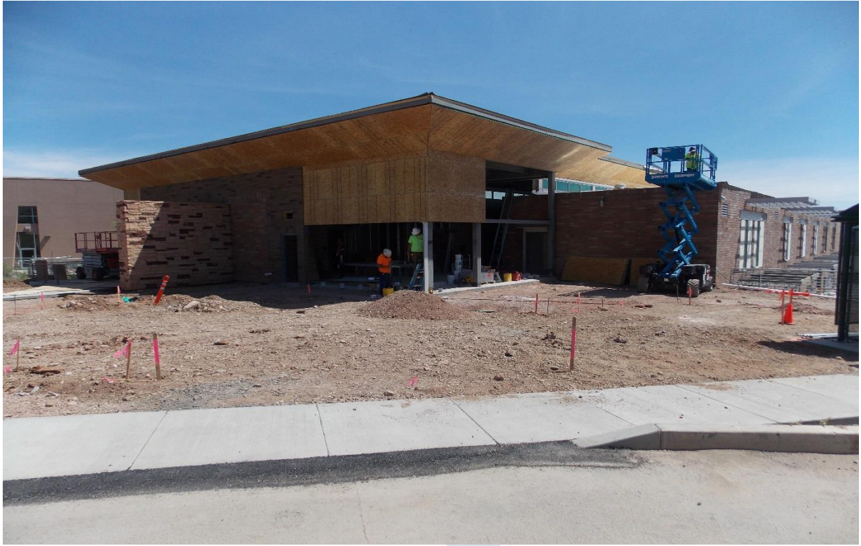
Installing Storefront Glass and Doors for New Front Entry
