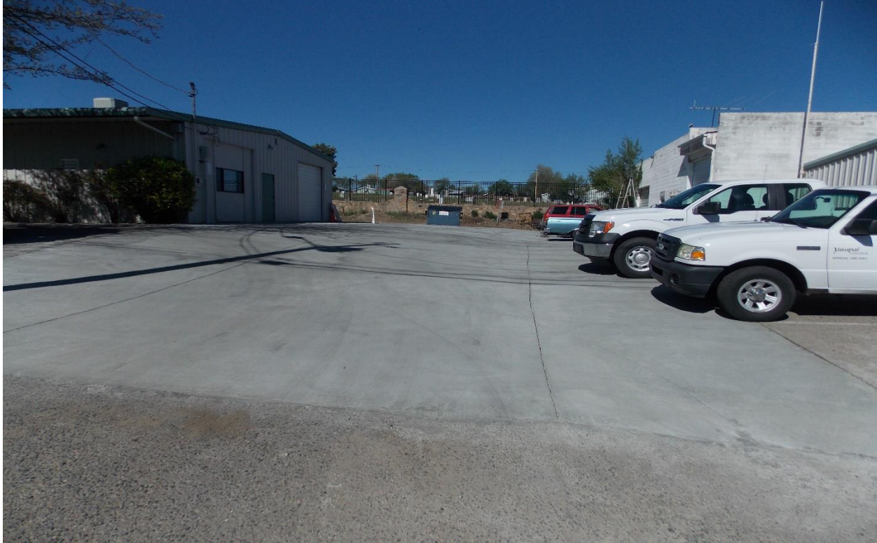
Building 20 Emergency Concrete Project
