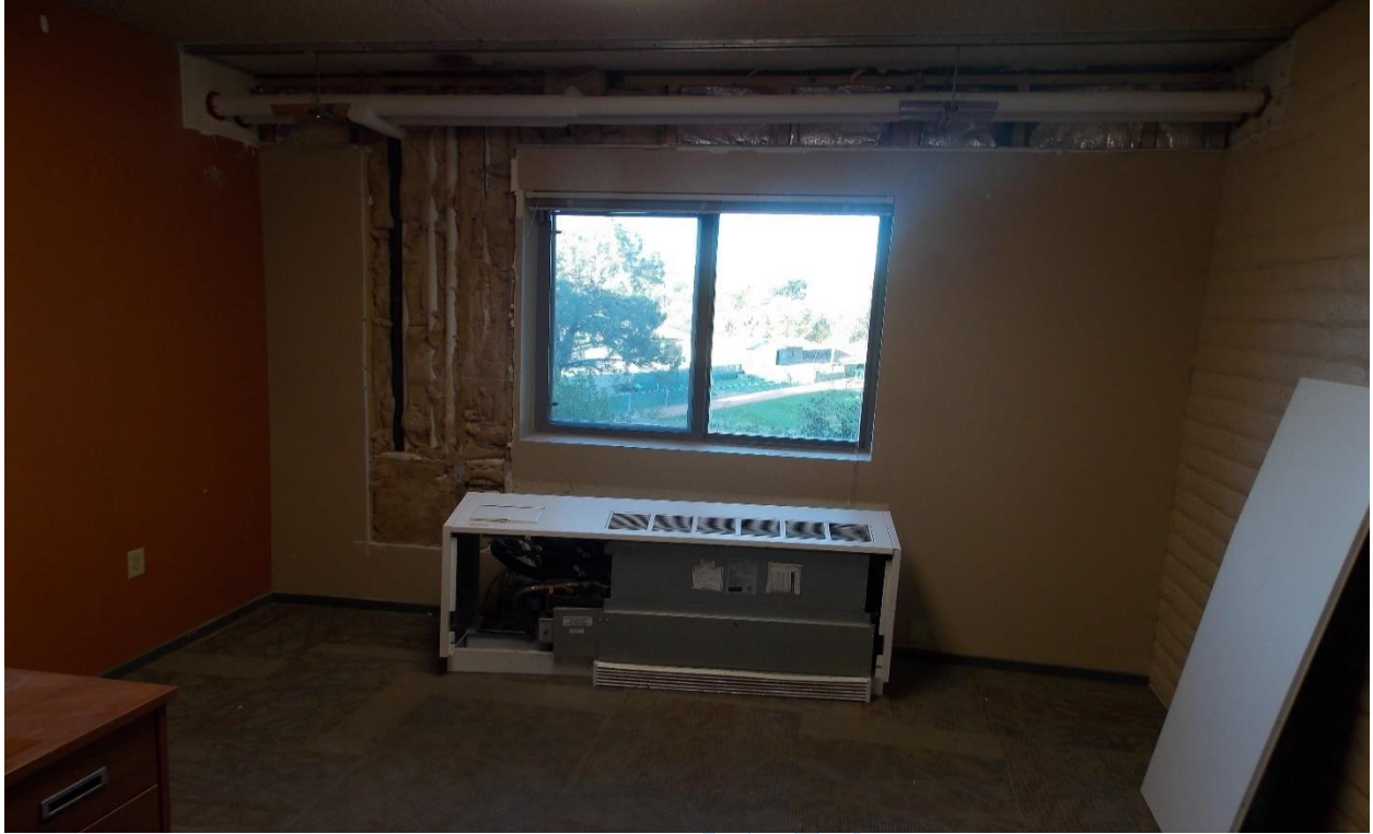
Typical Kachina Room Demolition in Preparation for New Piping (Facilities staff)
