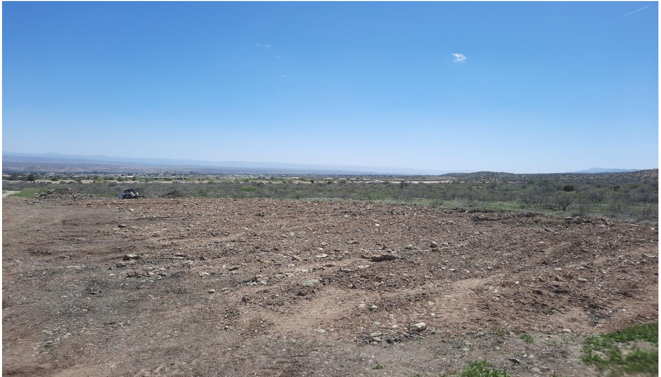
RV park construction activity east of the upper vineyard
