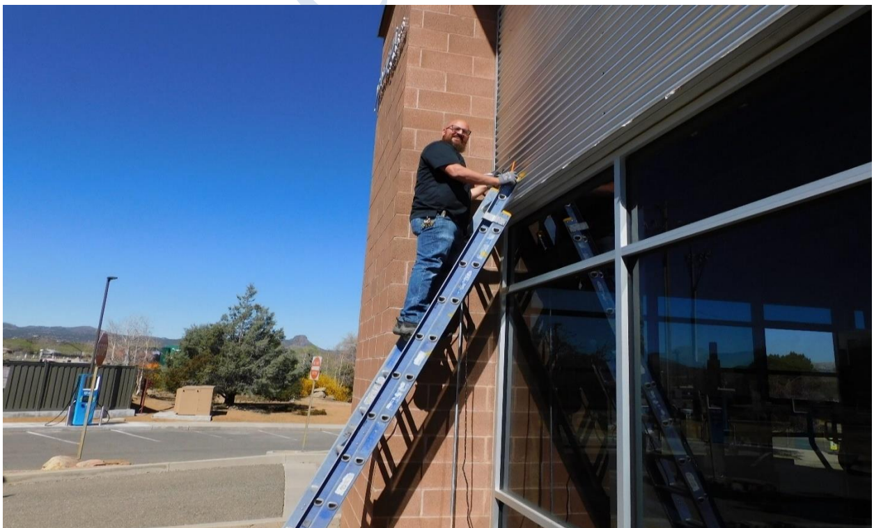
Electrical Supervisor Zack Vannoy installing new electrical service to Building 28 offices
