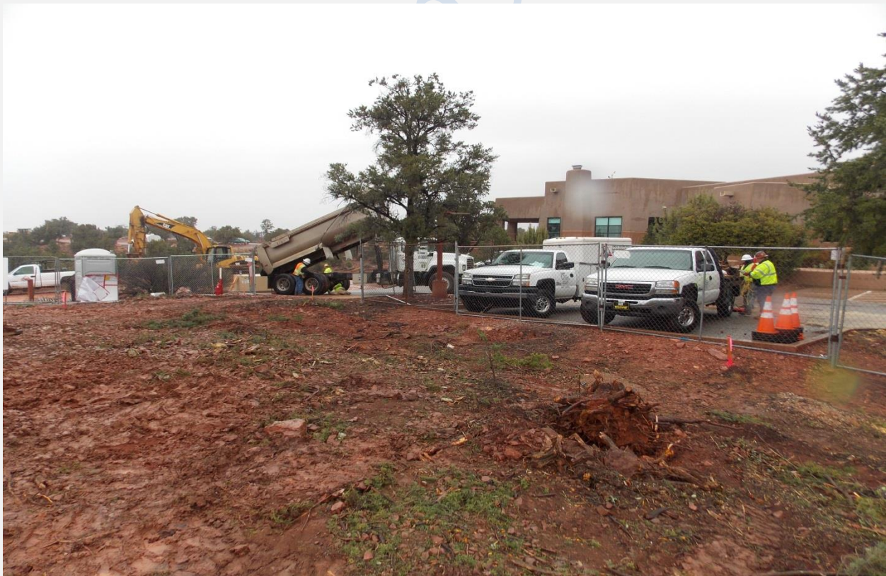
Site Clearing of New Sedona Center Lot
