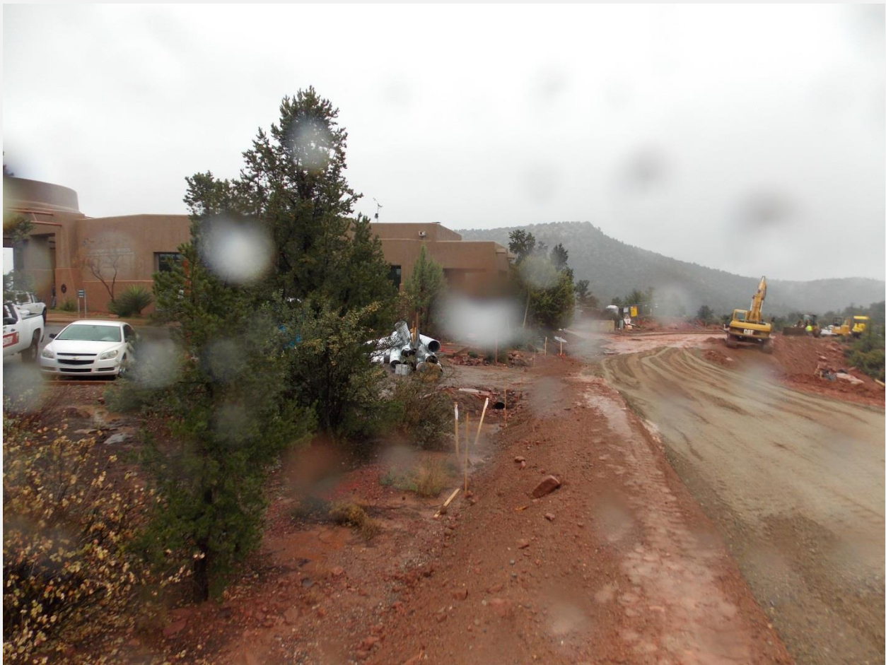
Road Base Being Installed on a Very Wet Day
