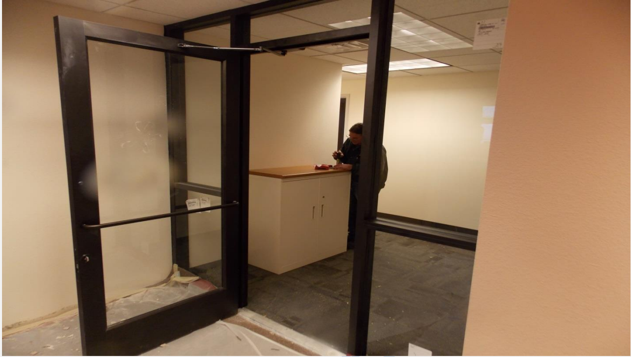
Entry to New IER Office Suite Building 32
