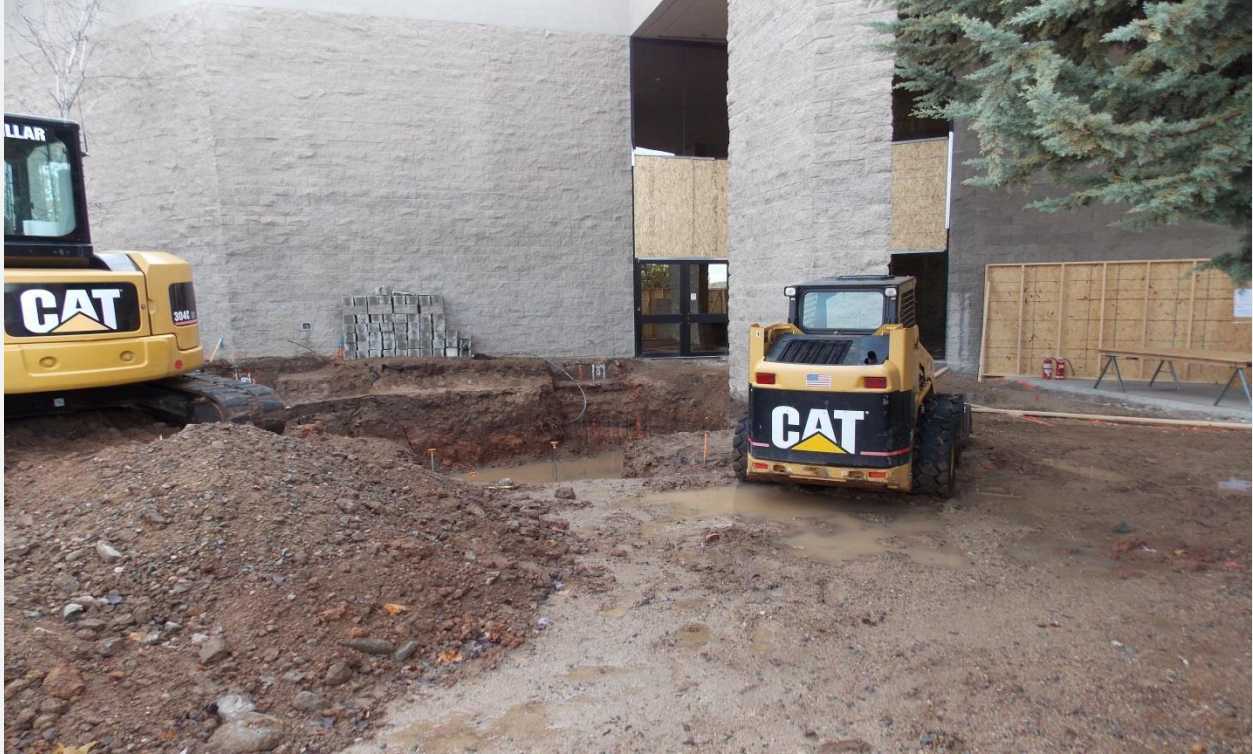
Location of New Elevator Shaft
