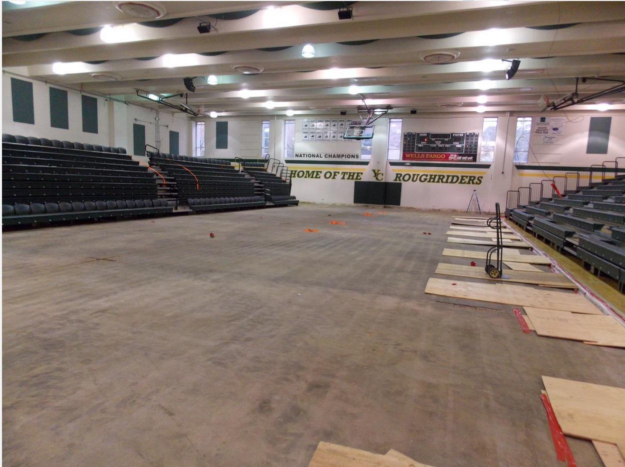
Ongoing Preparation for Replacement Gym Floor
