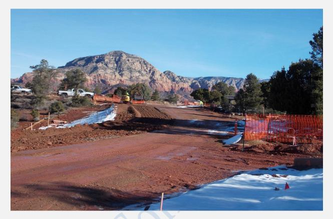
Installation of Storm Water Drainage and Retaining Wall Arts Village Drive
