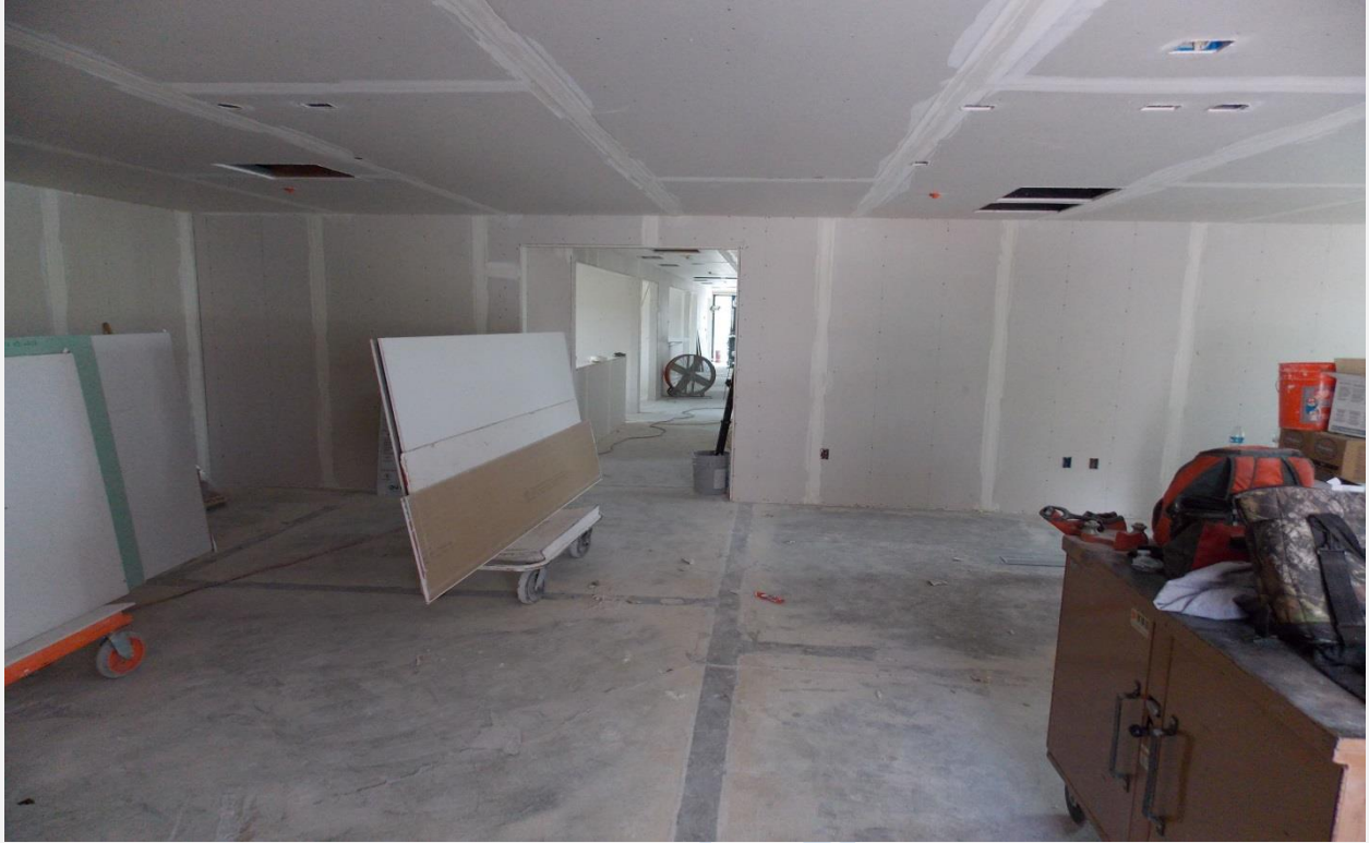
Building 31 Life Long Learning East Classroom
