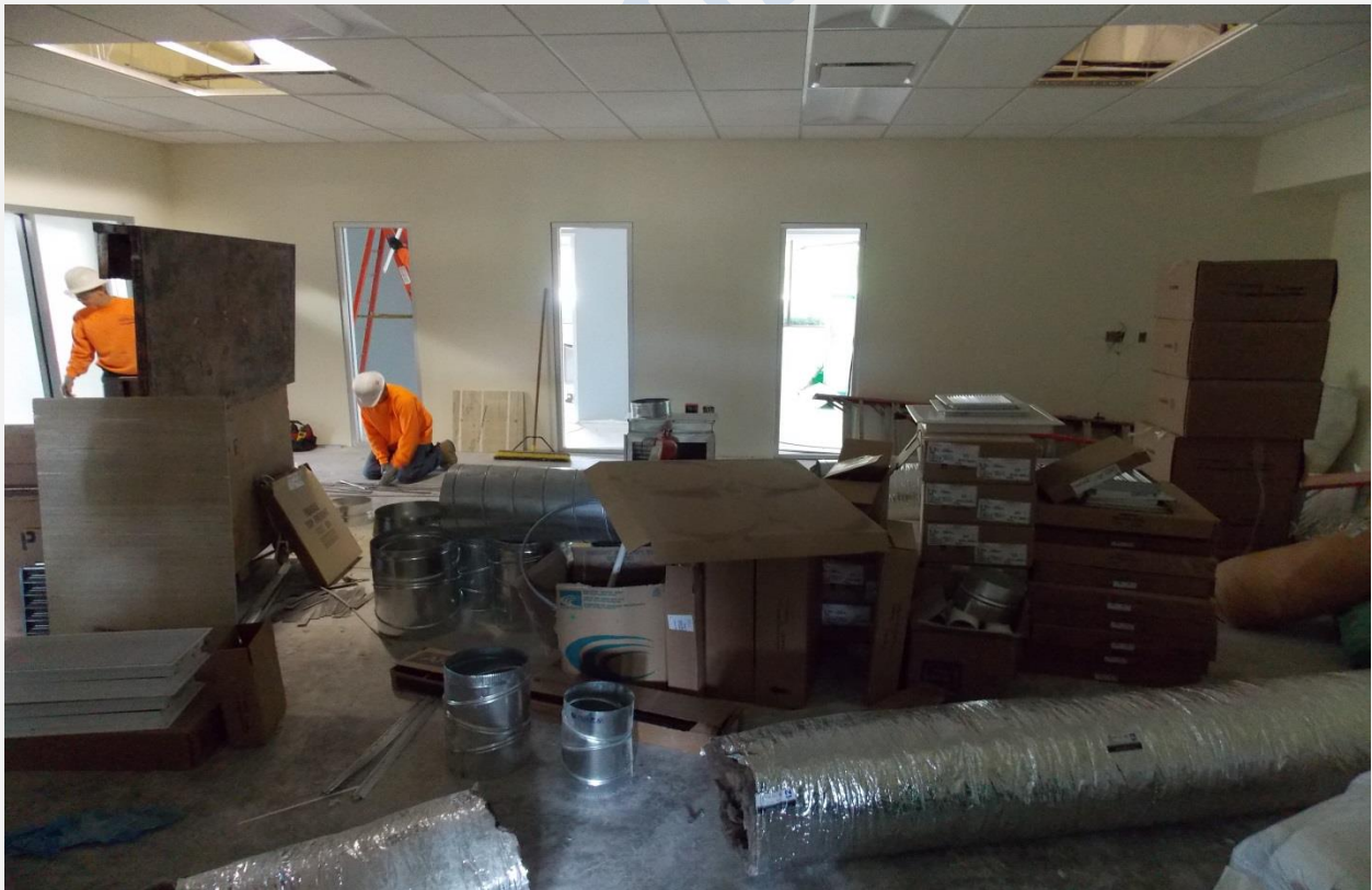
Building 29 REDC/Lifelong Learning Joint Use Multi-purpose Room
