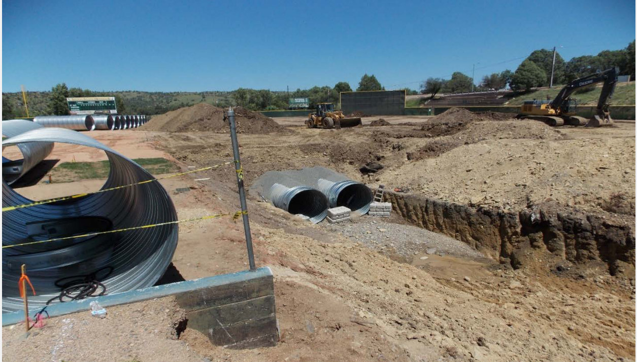
New Double Culvert Pathway under Baseball Field
