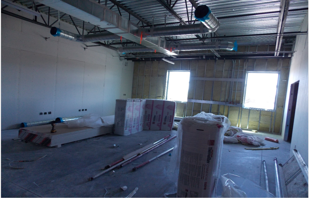
Installing Ductwork in New Classroom
