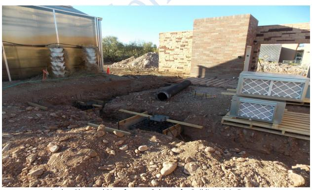
Anchor Plate and Piers for new Columns for Building Main Entrance
