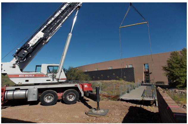
Lifting of Bridge between Buildings L and M for Structural Reinforcement
