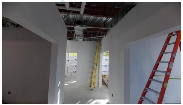
Installing Ductwork and Preparation for Ceiling Grid
