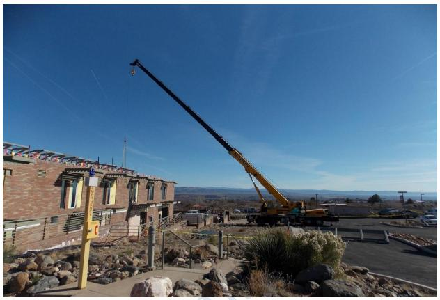
Setting Structural Steel for New Roof
