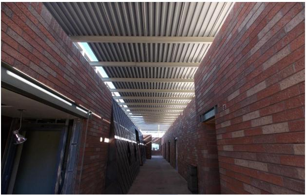
Roof Decking Enclosing Second Floor
