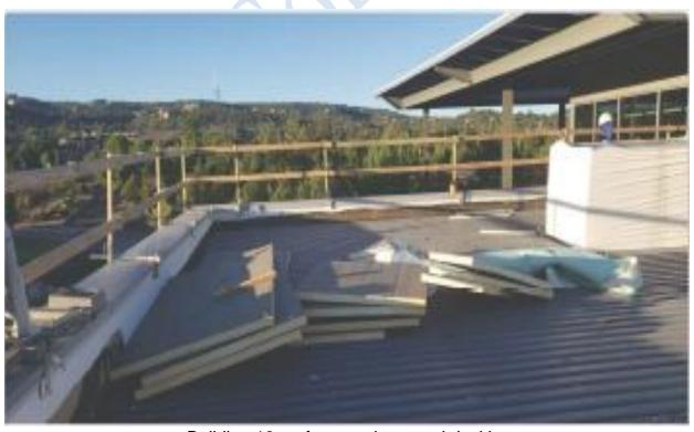
Building 19 roof removal to metal decking
