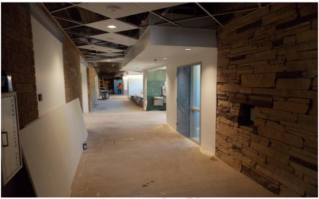
New ceiling and lighting being installed in the first-floor hallway
