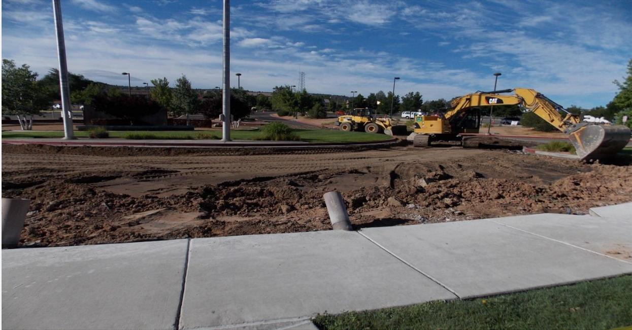
Replacing Damaged Asphalt with Concrete at Traffic Circle Prescott Campus
