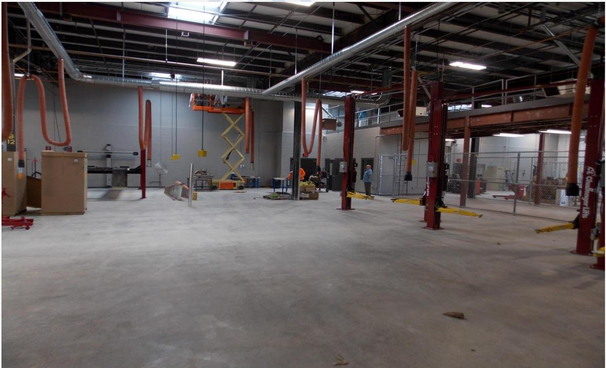
Exhaust Ventilation Installed Automotive Lab
