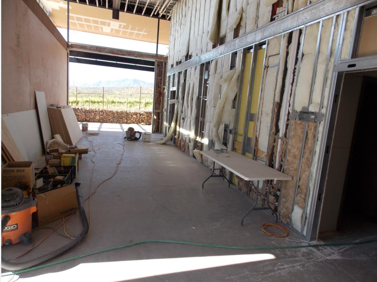
Tasting Room Framing and Insulation
