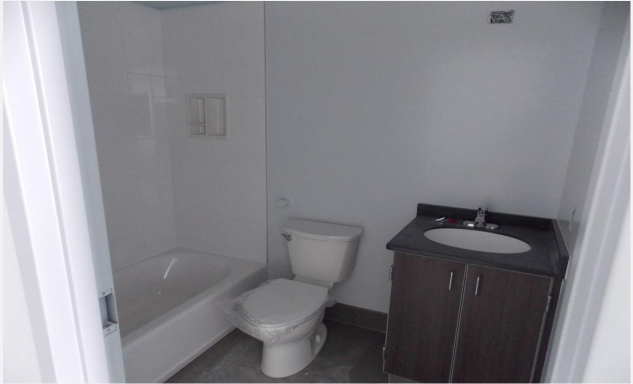
New Tile and Bathroom Fixtures
