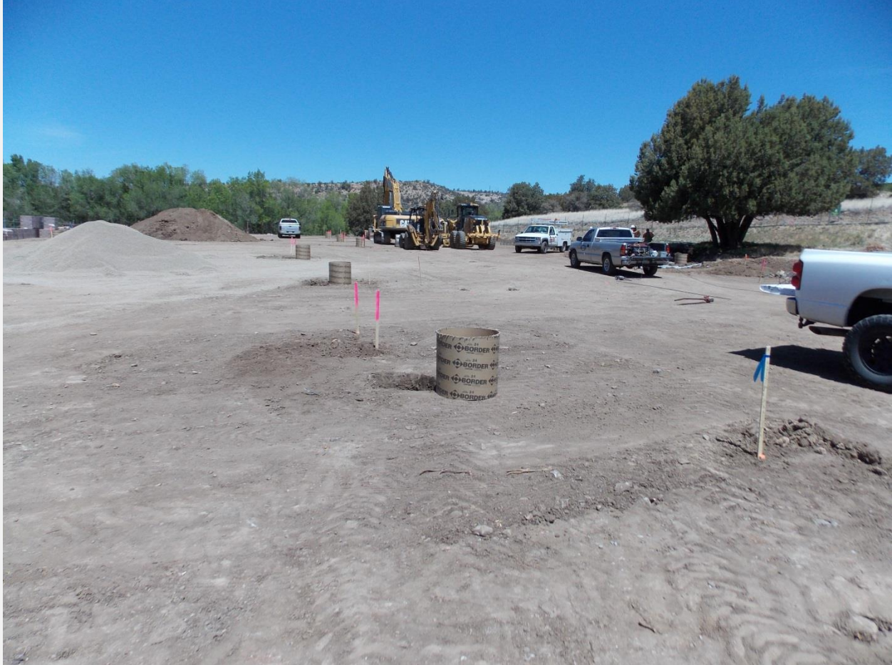
Boreholes for New Light Pole Bases
