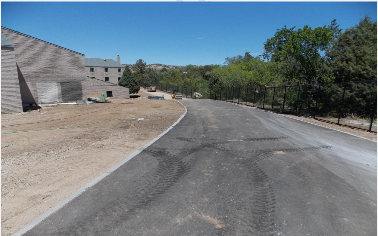
Fire Department Access Road and New Fence
