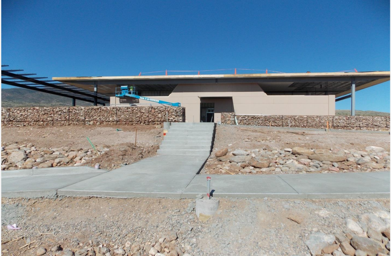
Gabion Wall Construction and Walkway/Access Ramp
