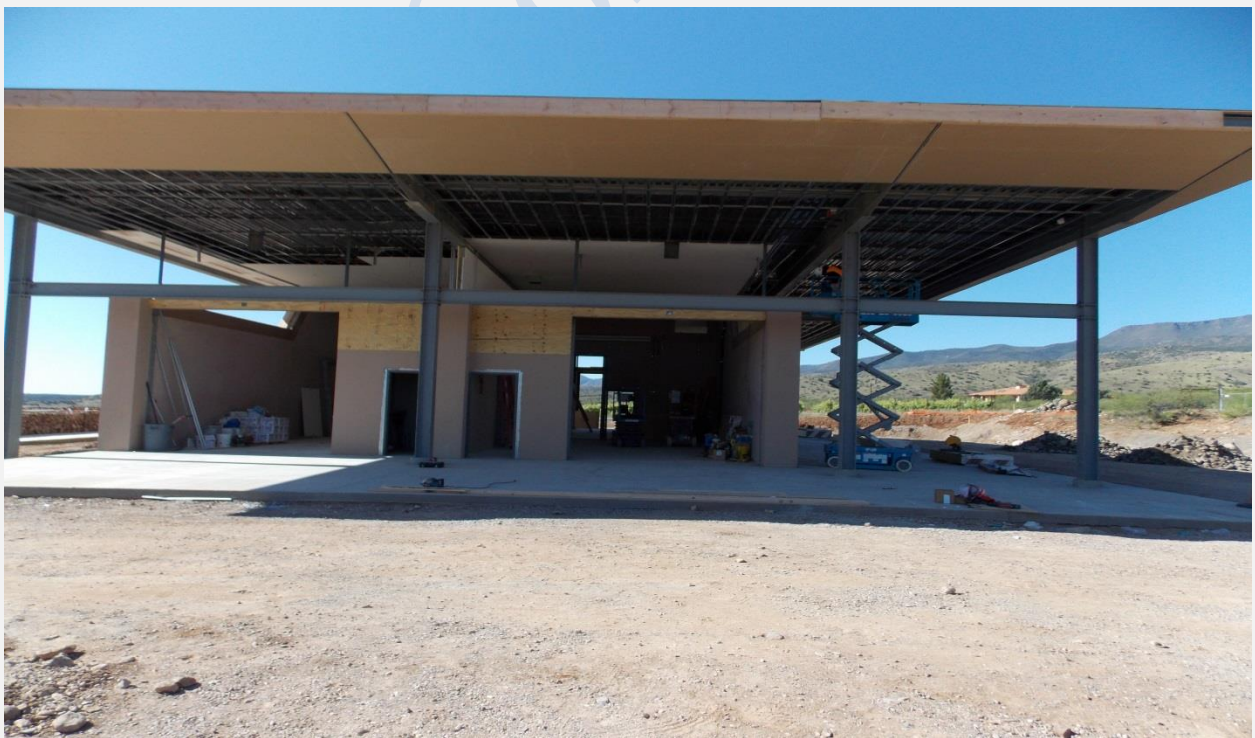
Soffit and Fascia Board Installation
