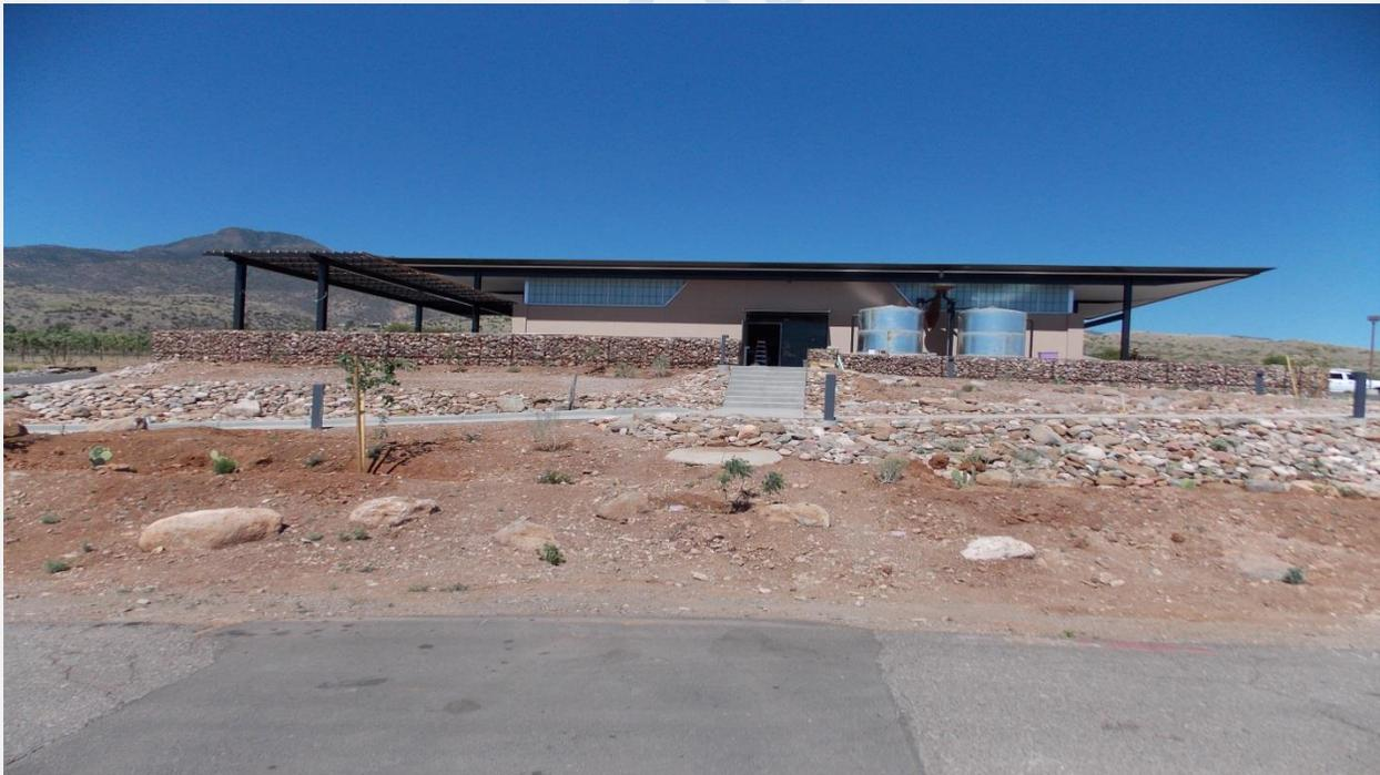
SWC East Elevation with Rain Water Capturing Storage
