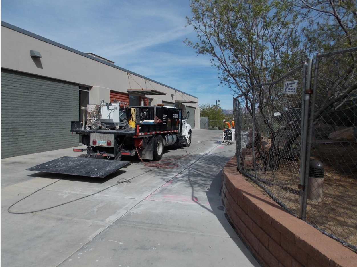
Concrete Sawing Between Buildings 2 and 3
