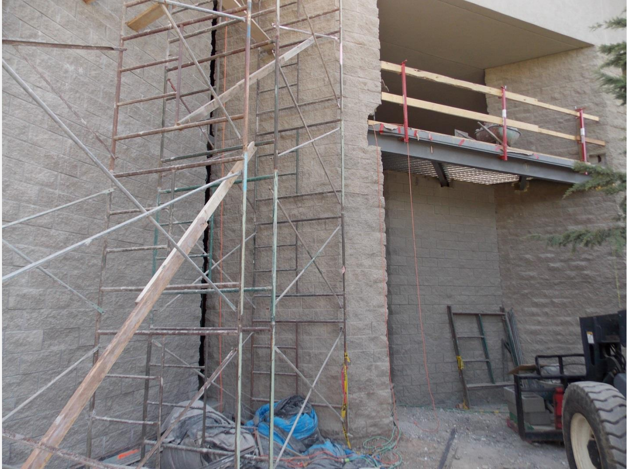
Installation of Steel to Support Second Floor Enclosed Balcony
