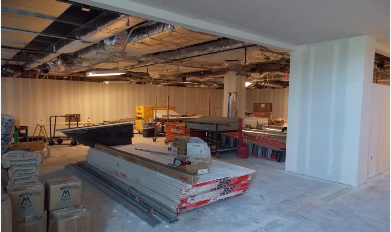
Building 3 Multipurpose Room
