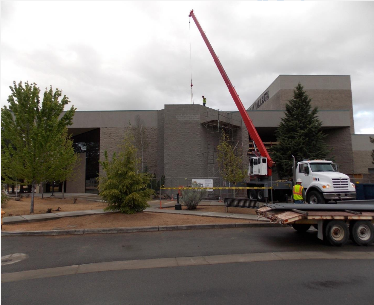
Installing Structural Steel for Elevator Shaft Roof
