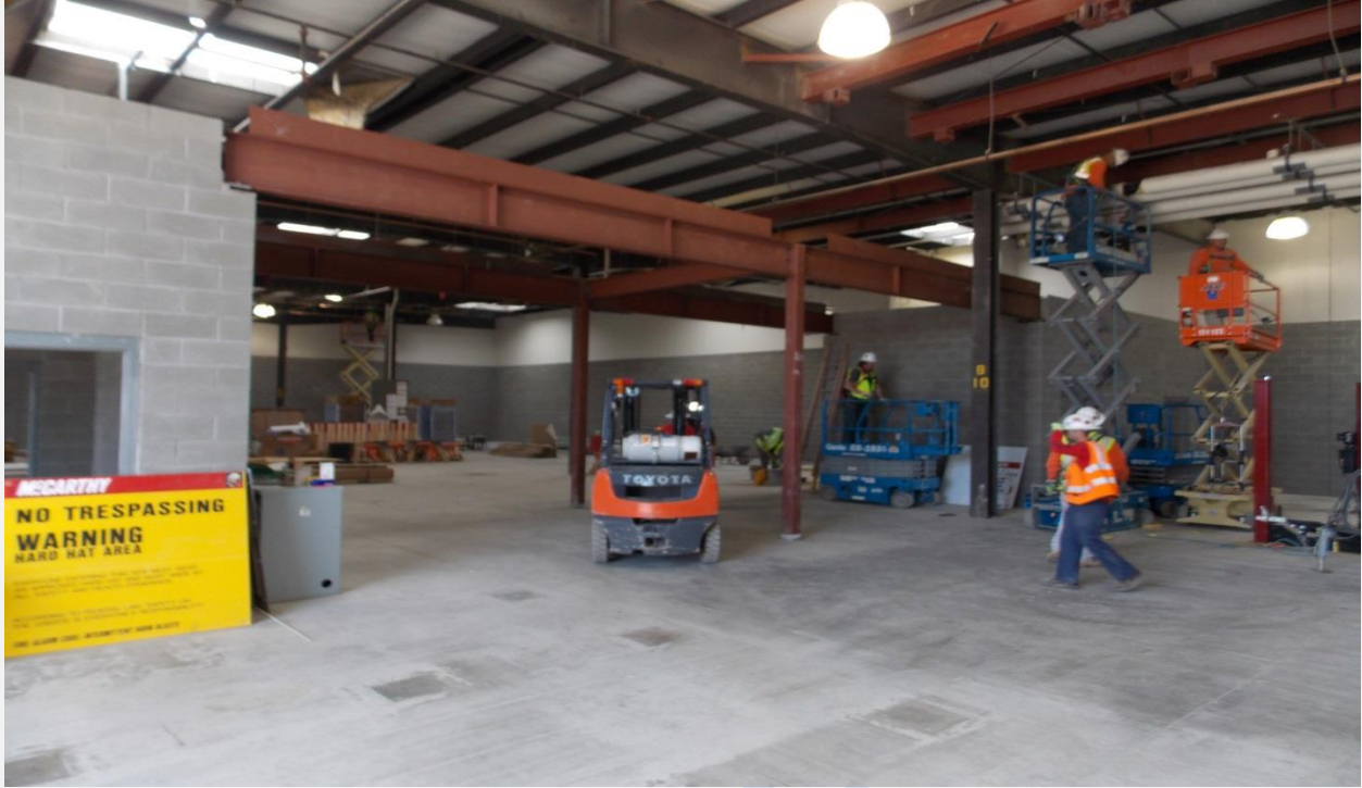
Structural Steel at Automotive/Diesel
