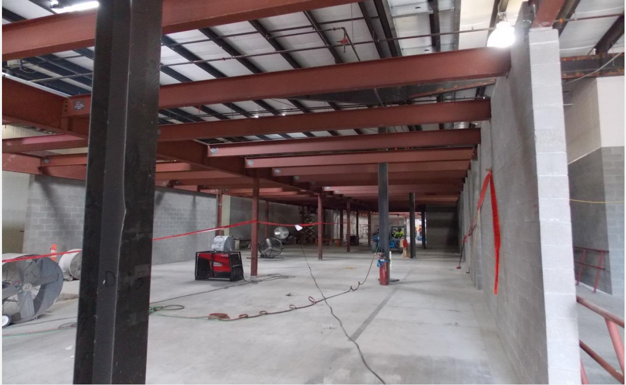
South Mezzanine Storage
