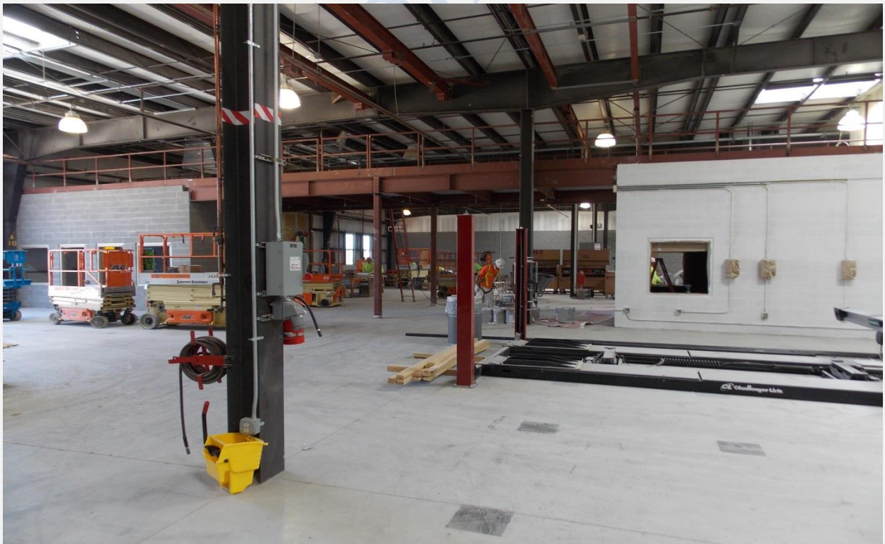
Mezzanine Storage Between Automotive and Diesel
