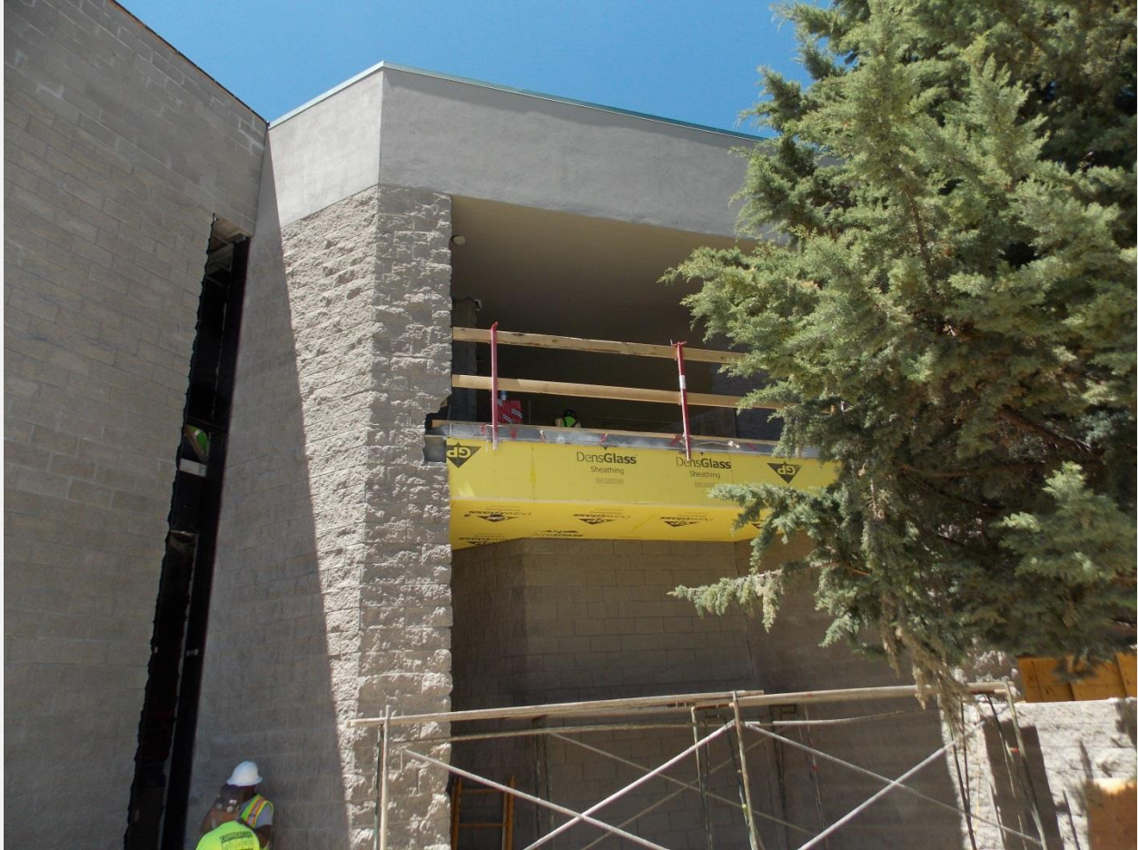
Enclosing the Second Floor Balcony
