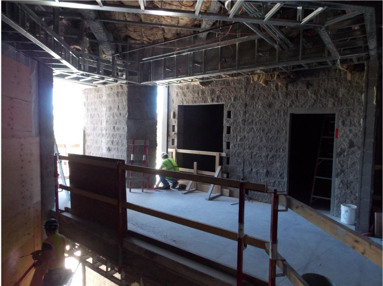
Installing Framing and Drywall at Second Floor Landing
