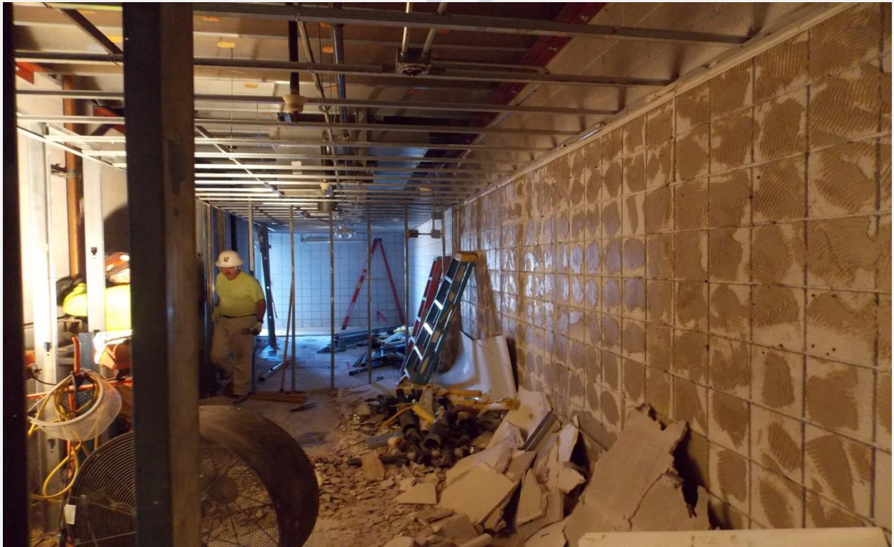
Renovating Space for Bluing Lab-Gunsmithing
