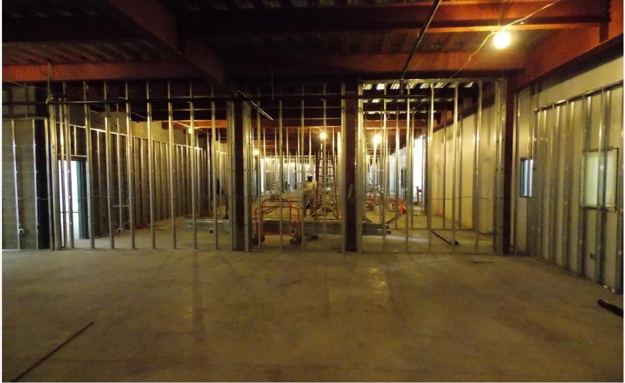
Framing of Walls for Classrooms and Computer Labs
