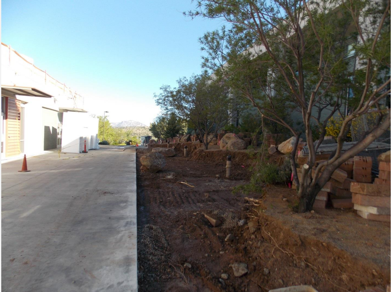
Site Preparation between Buildings 2 and 3
