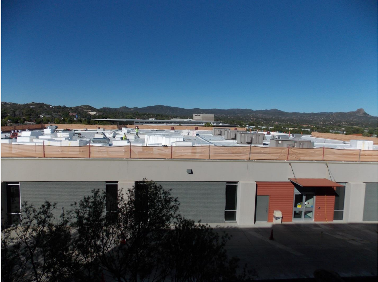
Building 2 Roof Replacement
