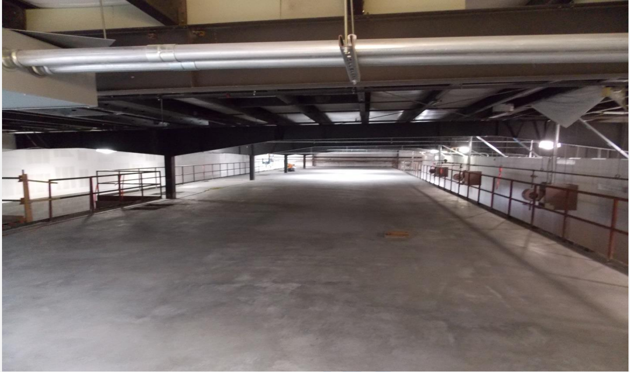
South Mezzanine Storage
