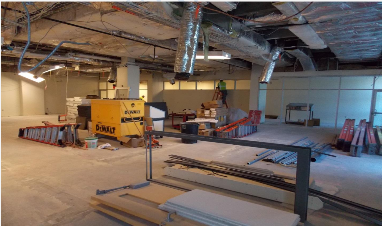
Building 3 Multipurpose Room
