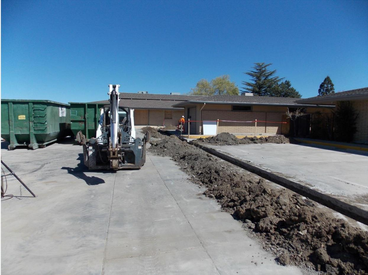
Trenching and Saw Cutting for Buildings 30 and 31 New Water Line
