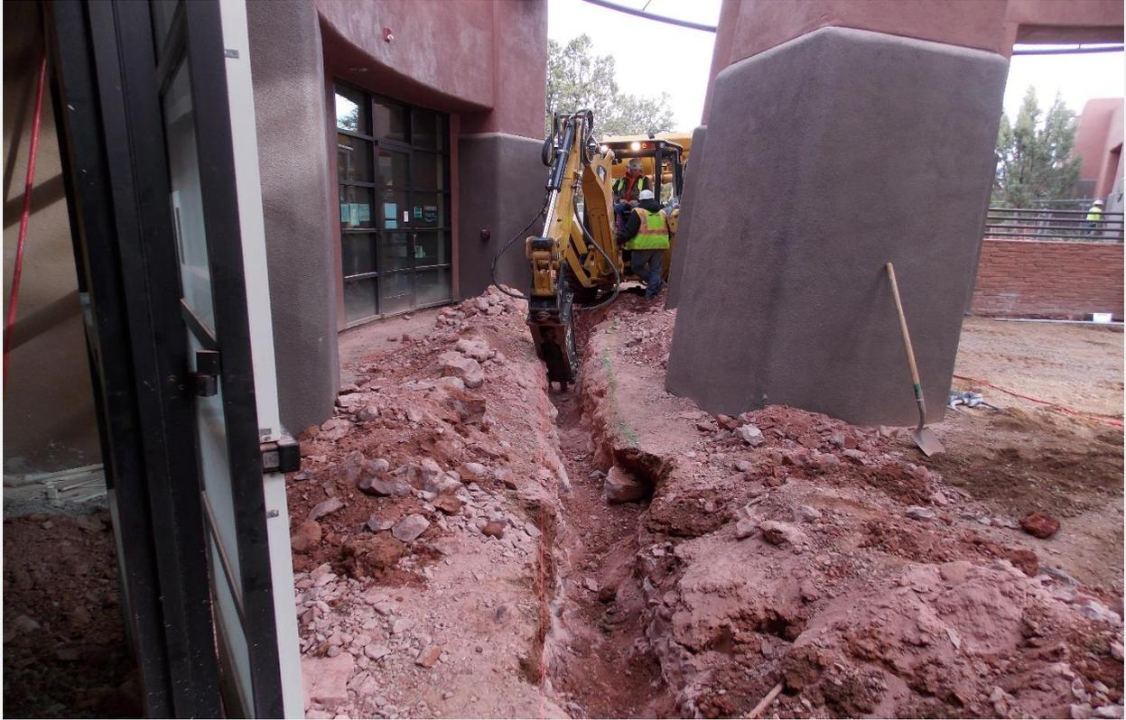
Use of 1,000 Pound Backhoe Hammer to Break Rock for Culinary Waste Grease Line
