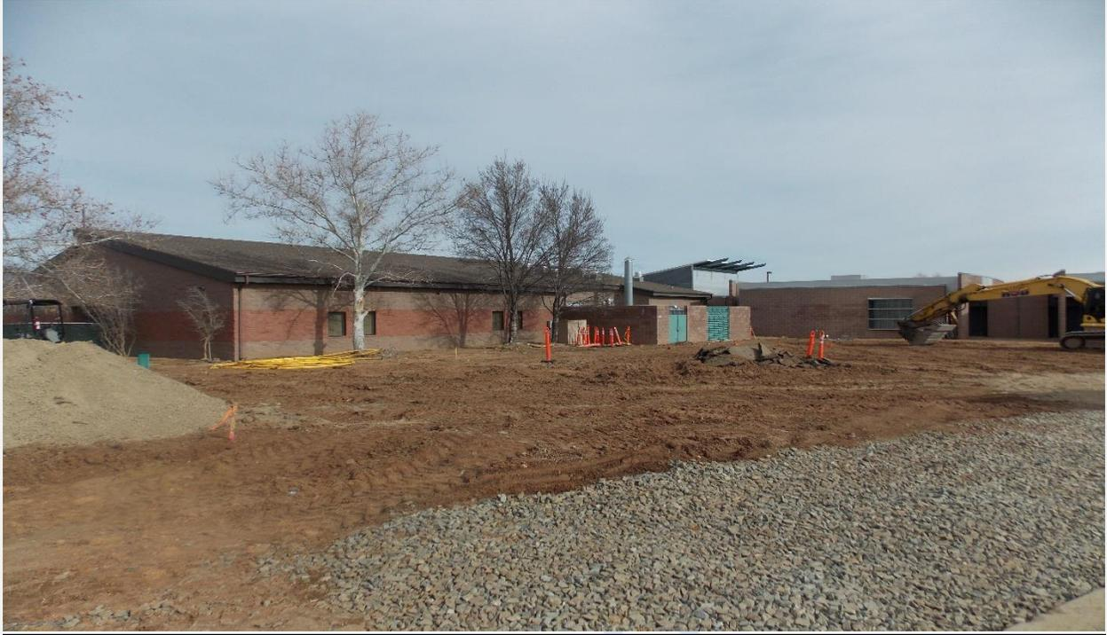
Installing New (Yellow) Gas Line for Central Plant
