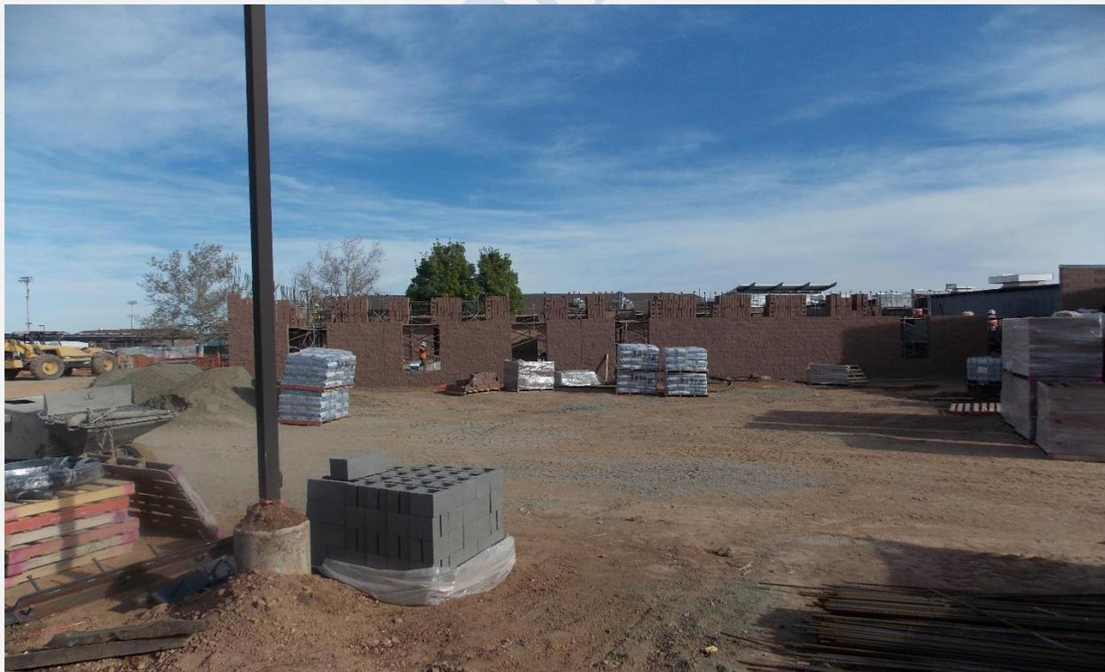
Masonry Exterior Wall Construction First Floor of Addition
