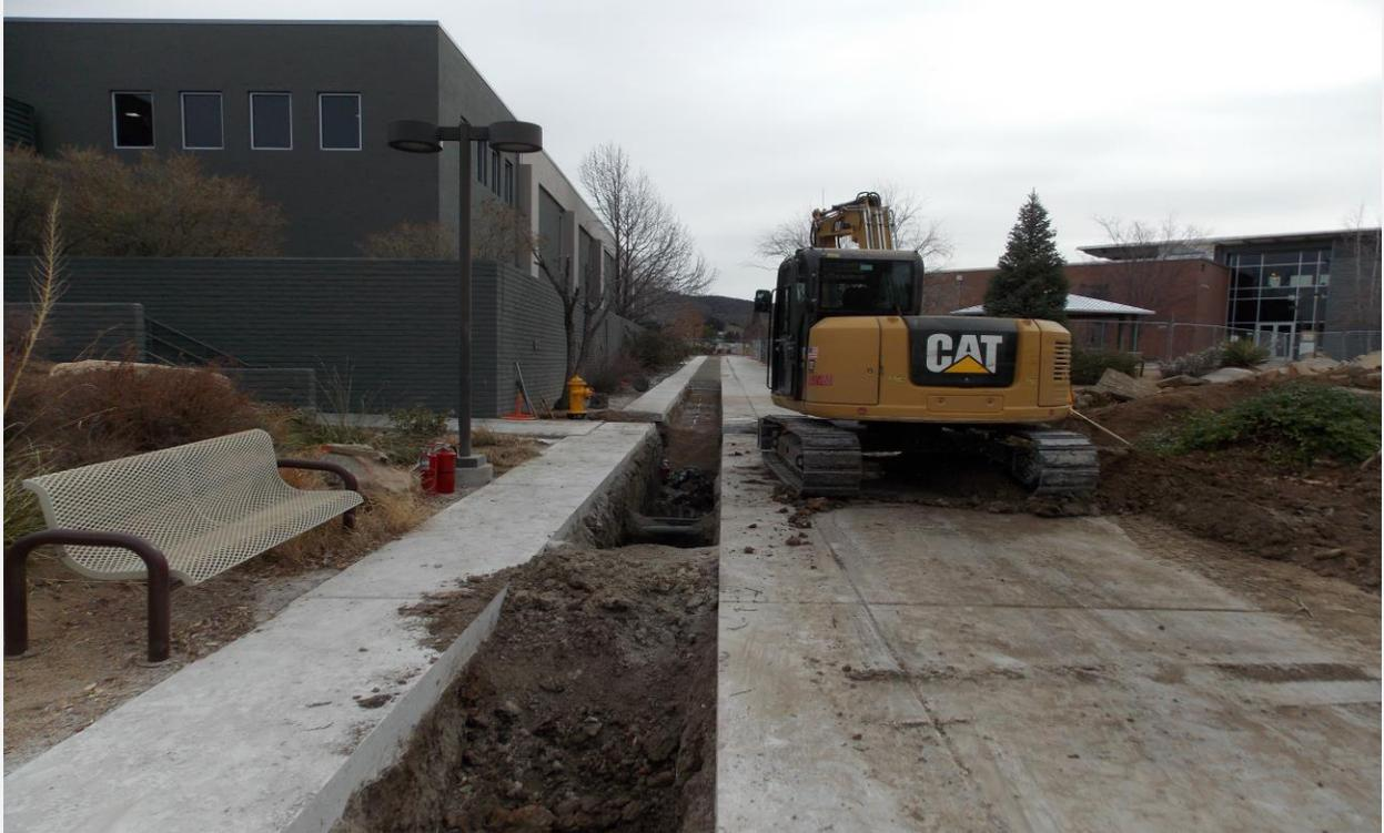
Backfilling Trench Between Buildings 2 and 19
