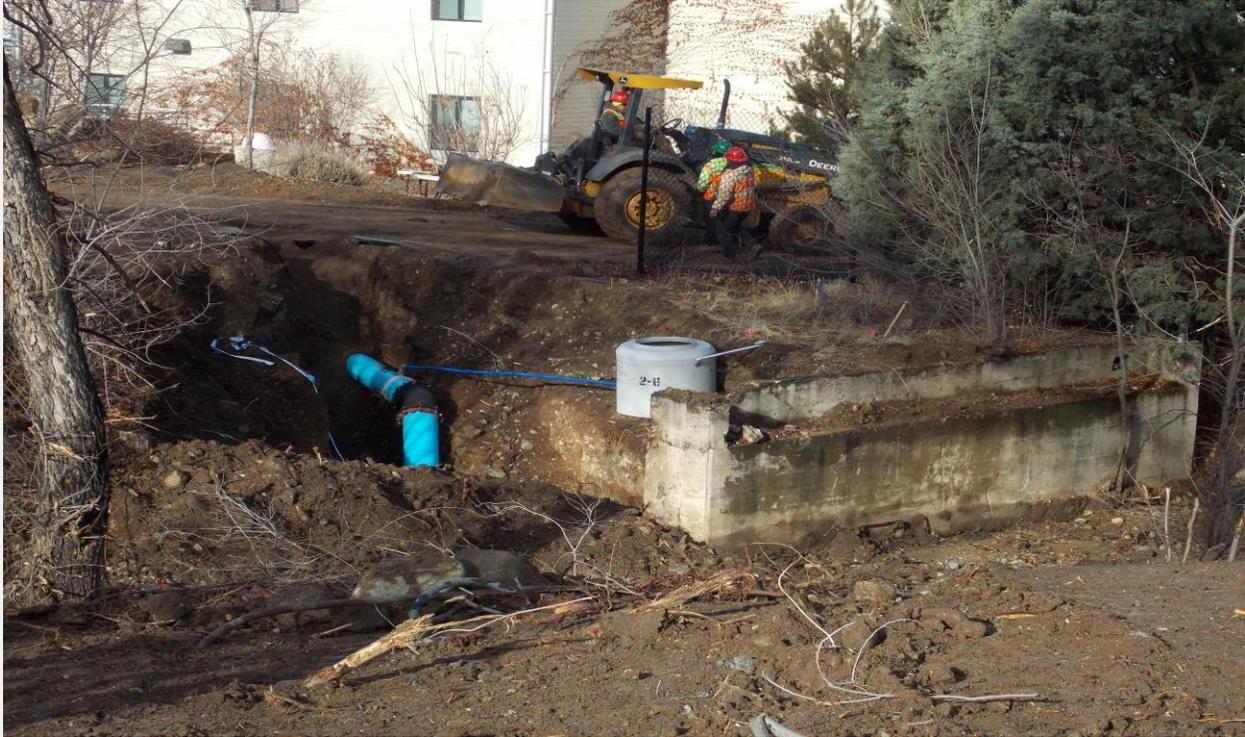
Installing New Section of Water line Near Marapai Hall
