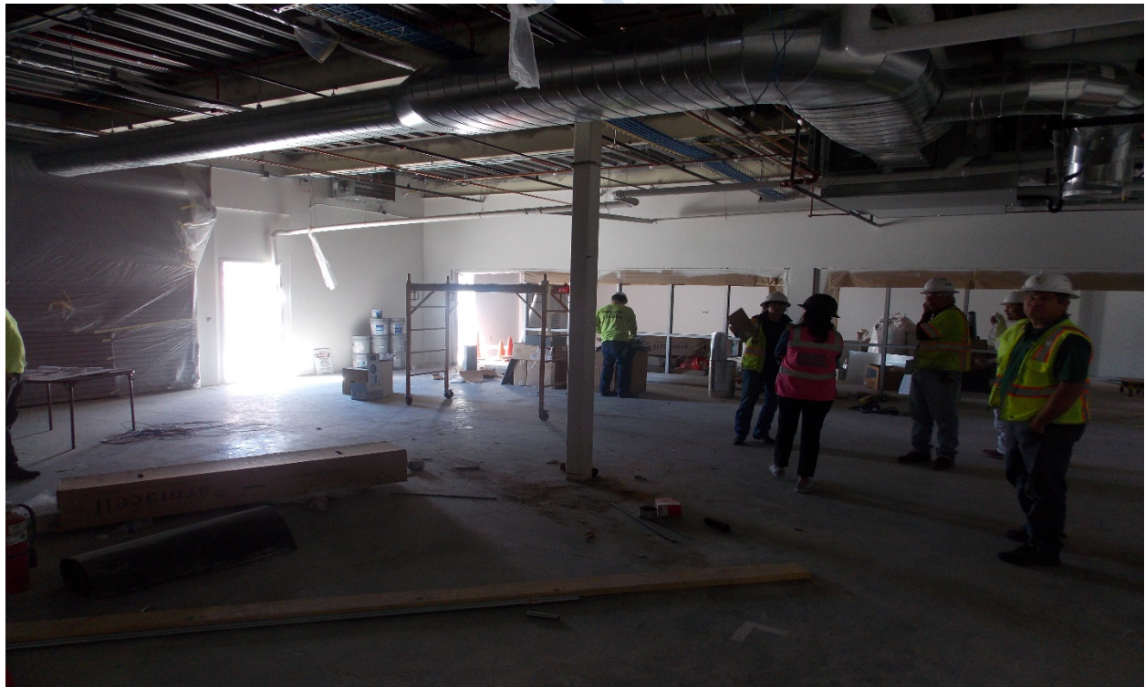
Advanced Manufacturing Lab looking towards the clean lab
