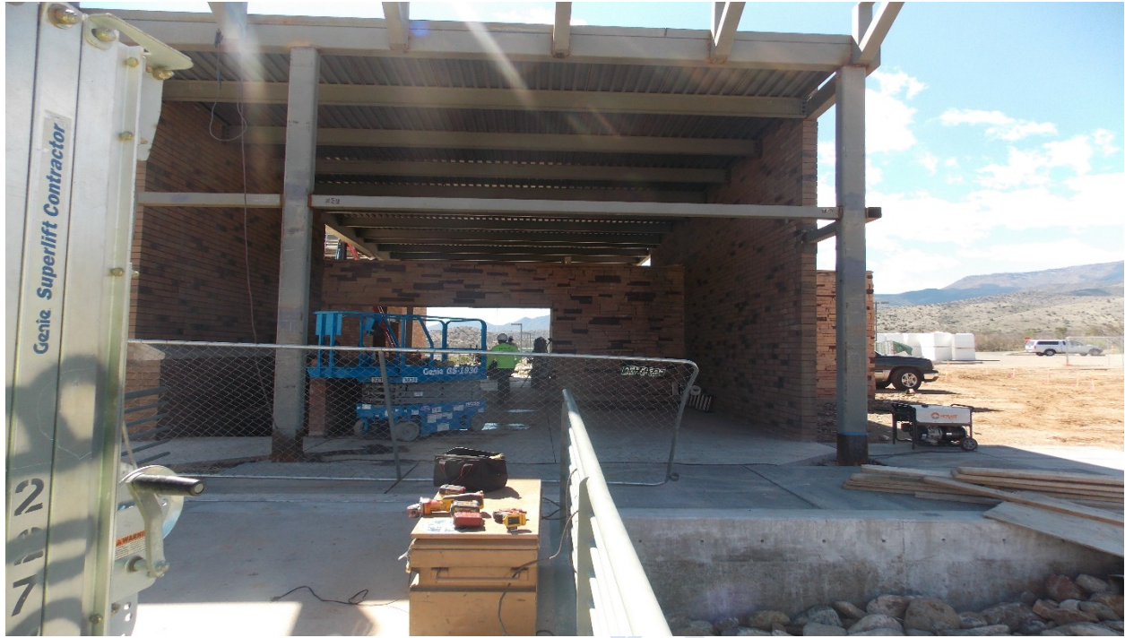
Building M side of the new front entrance
