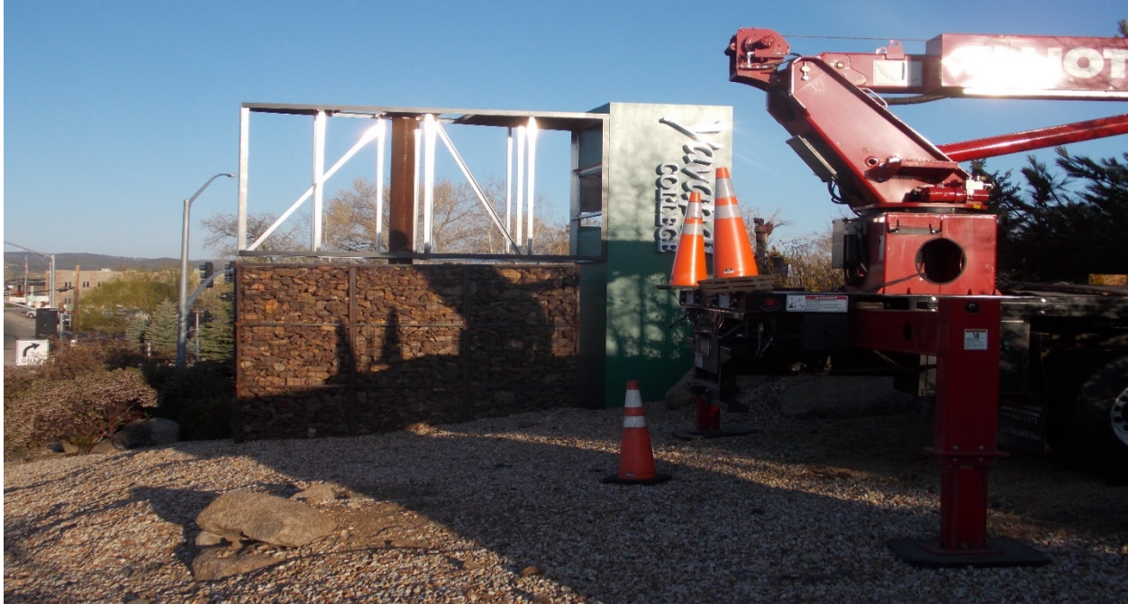
Install Marquee Structural Support
