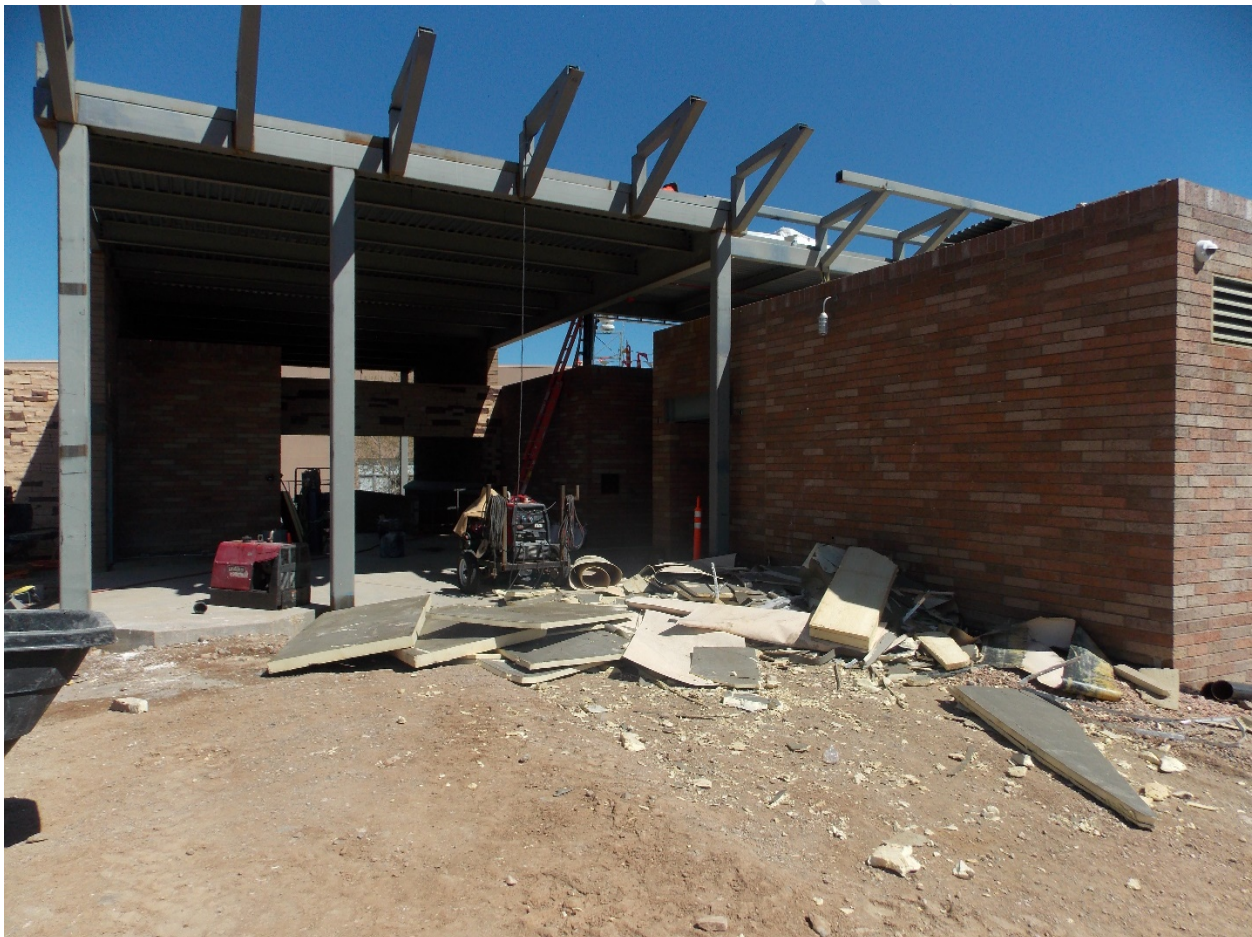
Steel in place for front entrance
