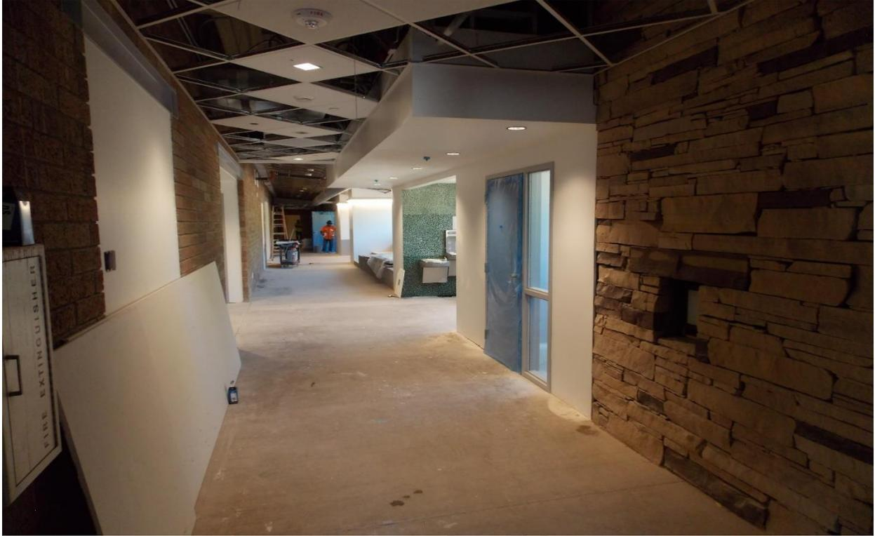
New ceiling and lighting being installed in the first-floor hallway
