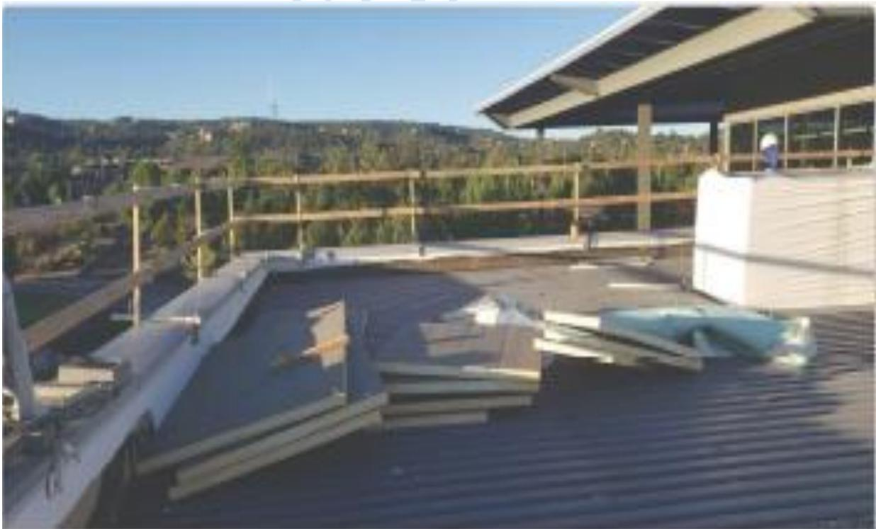
Building 19 roof removal to metal decking
