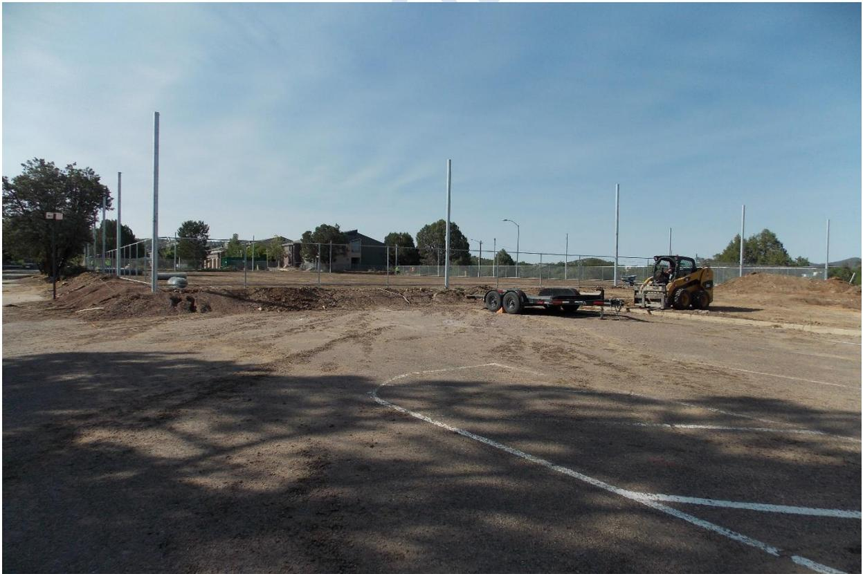
Installation of structural support for fence and netting system
