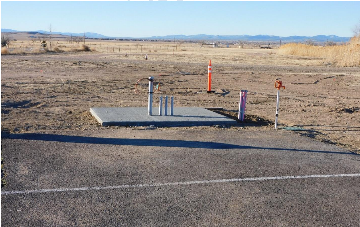
New electrical and water services
