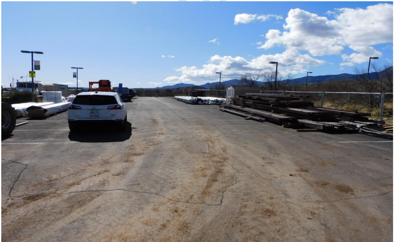
Engineered building components arrive on site
