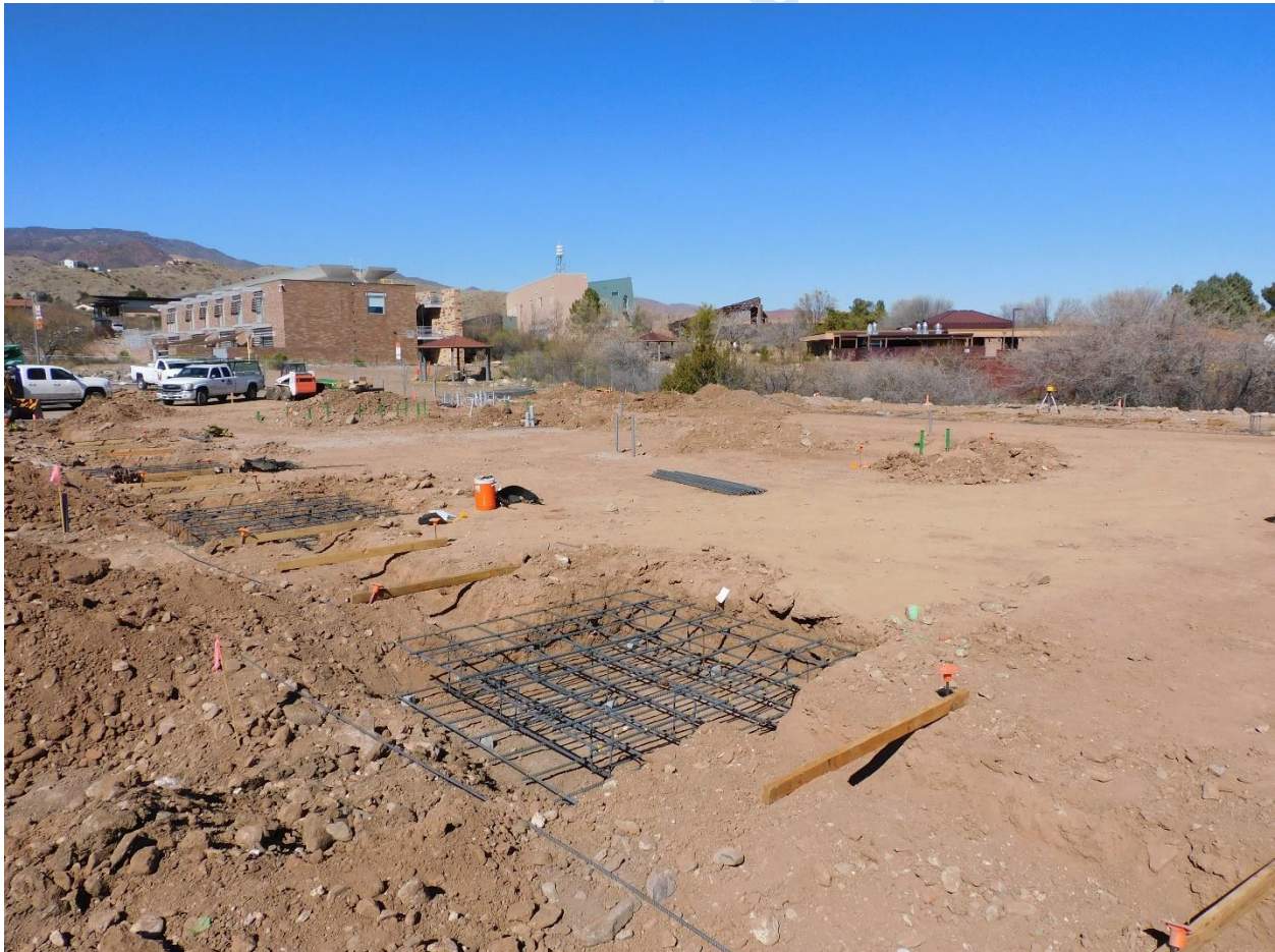
Location of new building column footings
