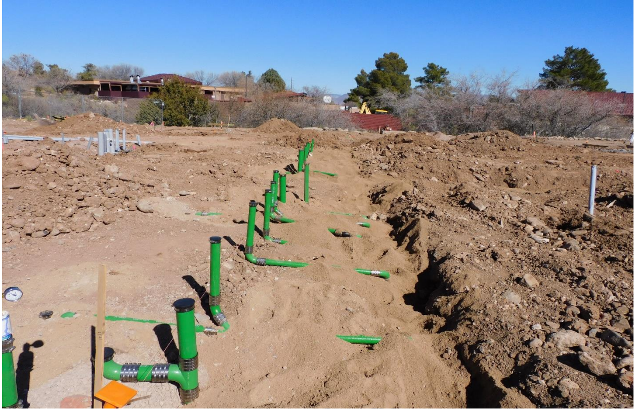
Plumbing underground stubb outs
