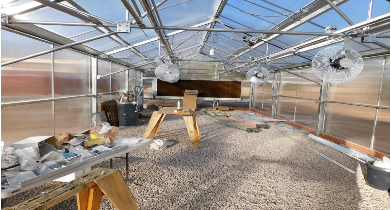
Installation of fans and other electrical items
