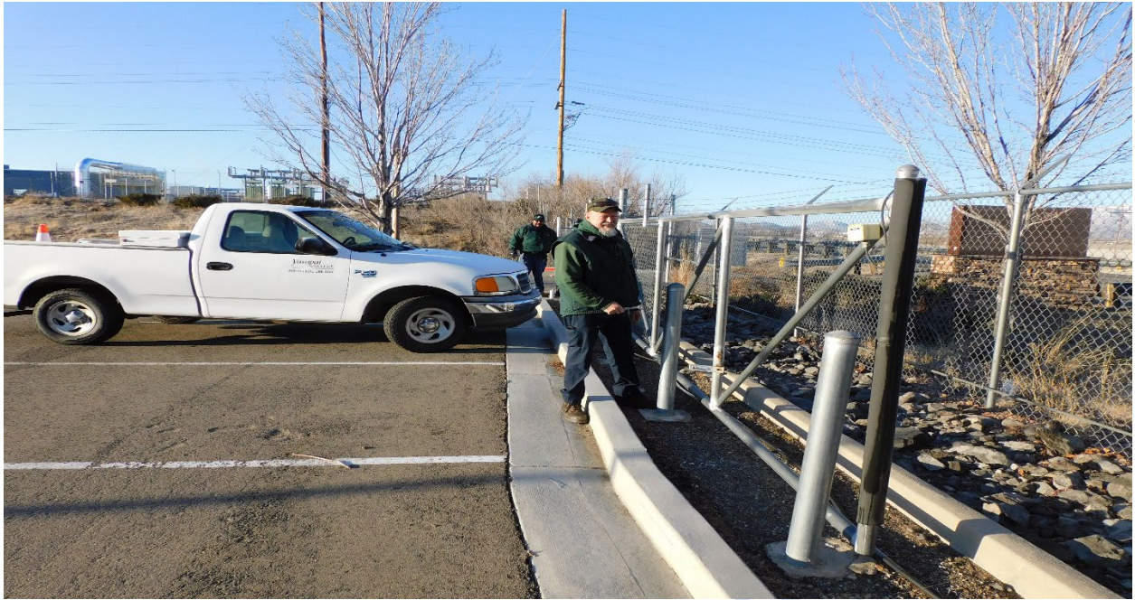
Auto Technicians Wade Milner and Roy Frias repairing the vehicle gate at CTEC
