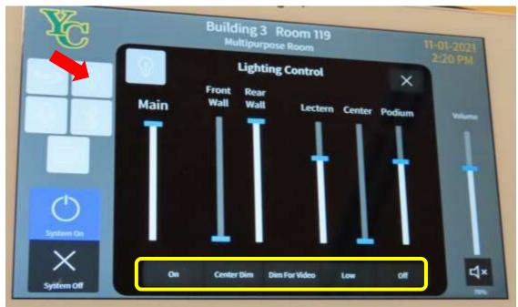
The options along the bottom of the screen automatically adjust the room lights for most situations:
