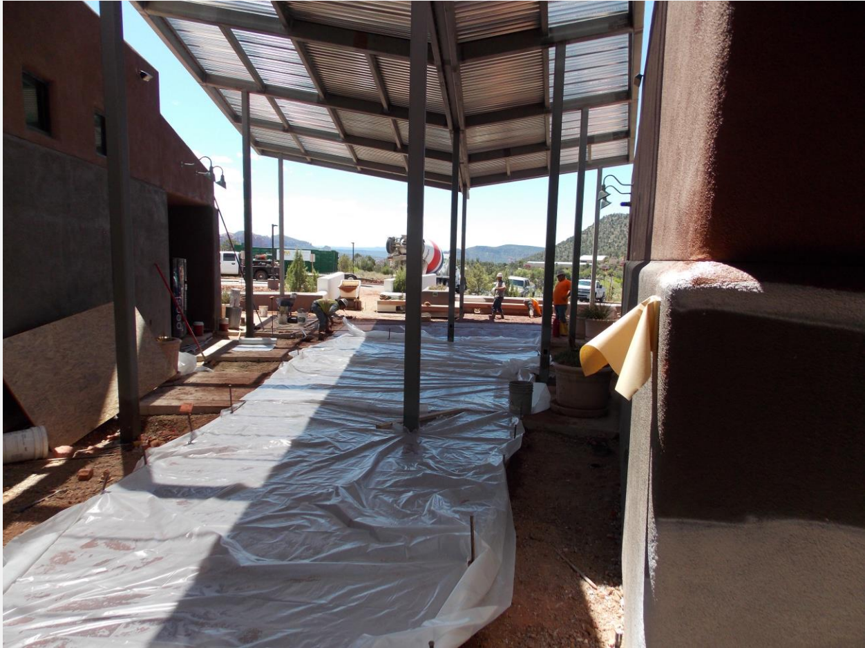
Preparing New Front Entrance for Colored Concrete
