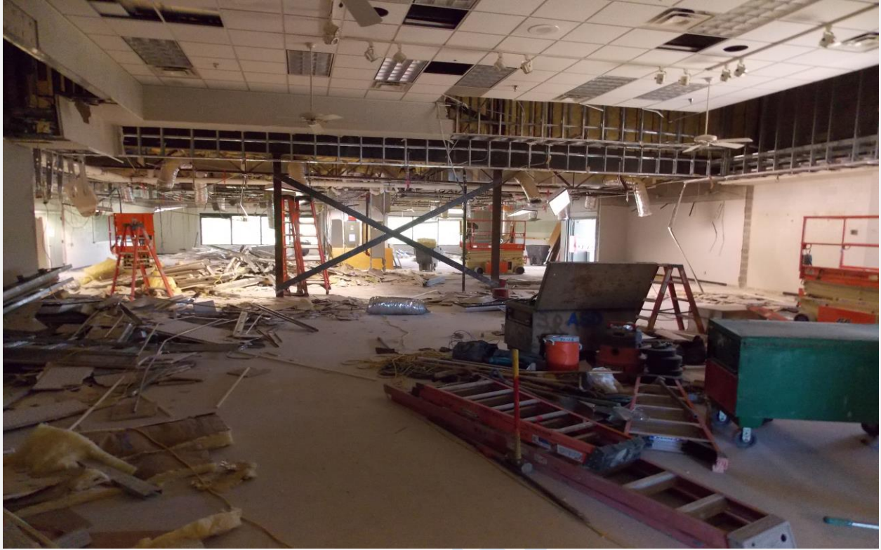
Building 15 Second Floor Demolition
