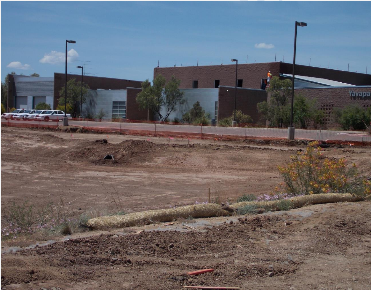
Parking Lot Grading with the Building Addition in the Background
