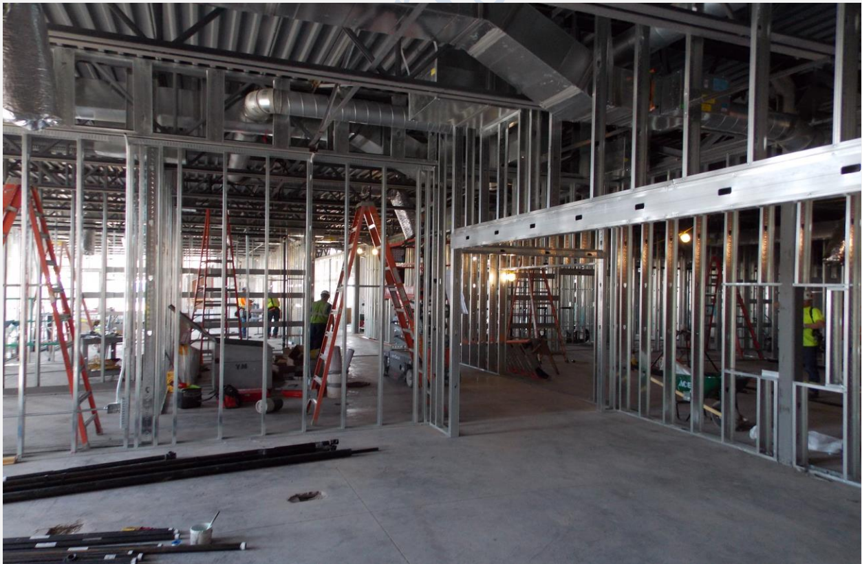
First Floor Framing HVAC Install and Fire Sprinklers
