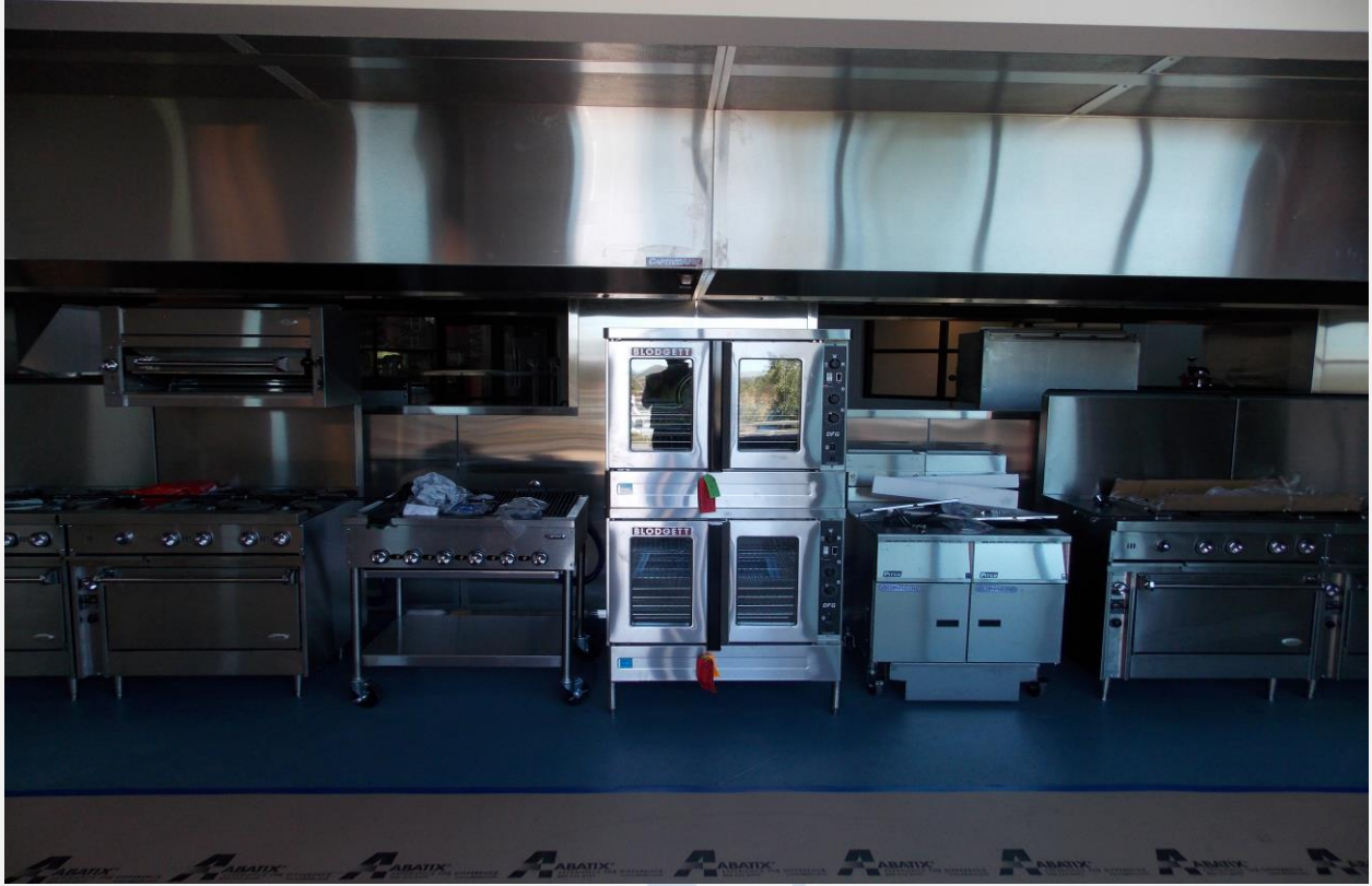
Setting Kitchen Equipment in Culinary
