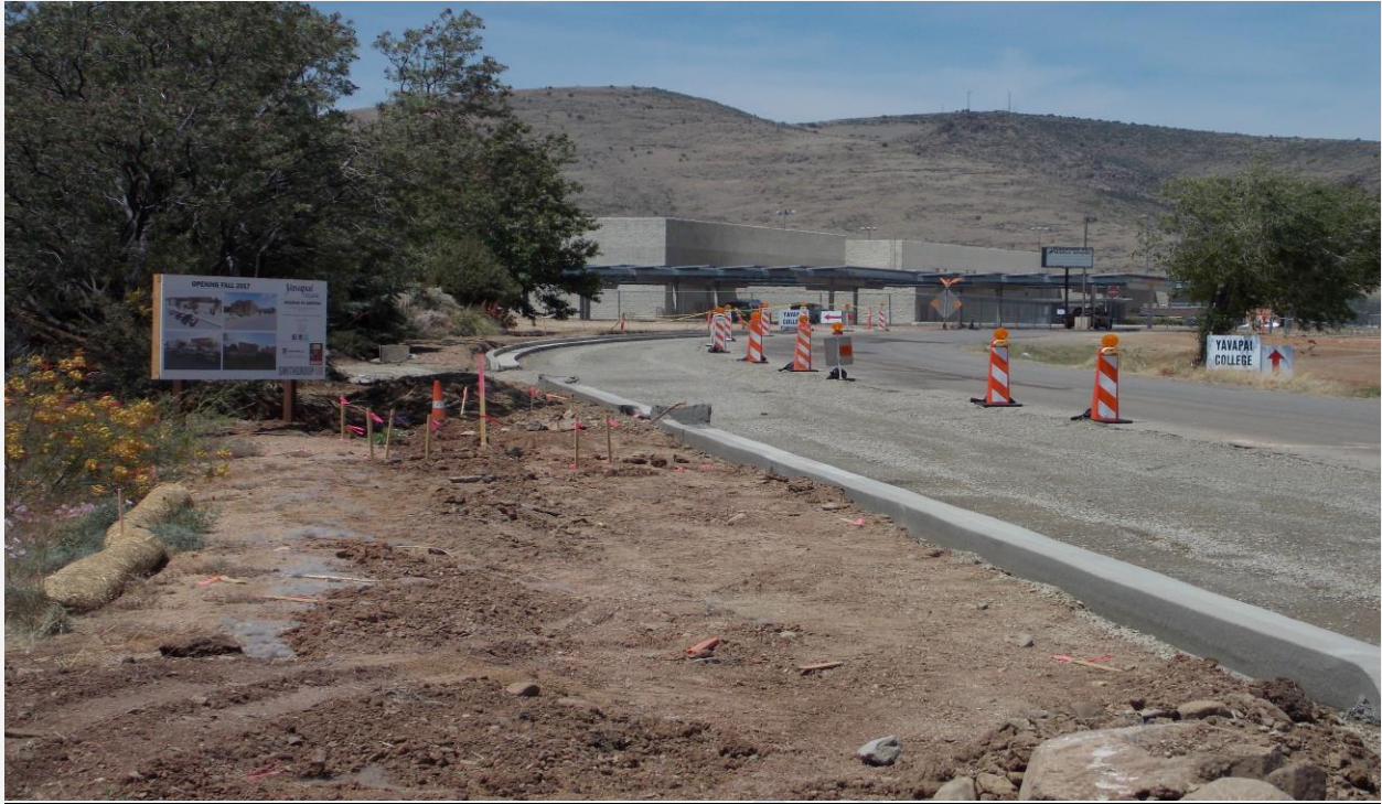
New Curb and Gutter and Sidewalk Preparation at Panther Path
