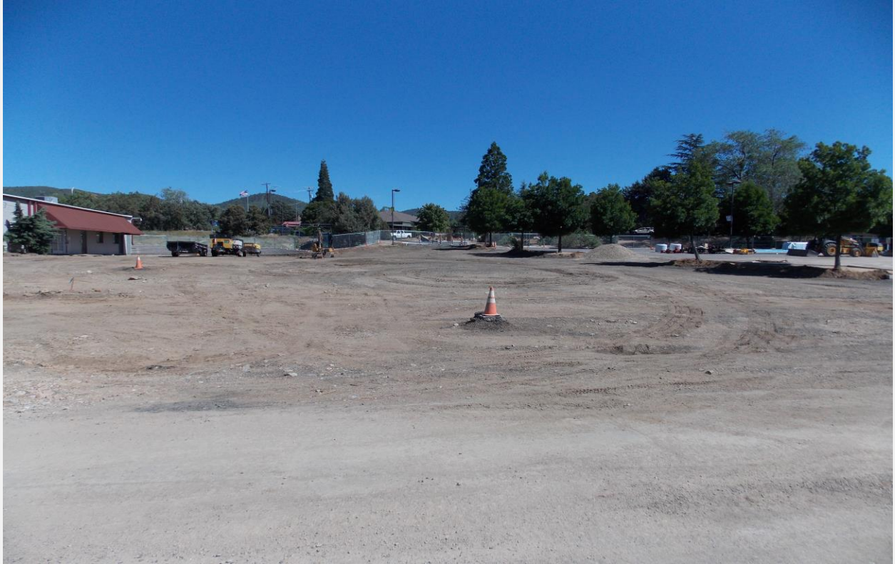
Building 7 Parking Lot and Water Line Replacement
