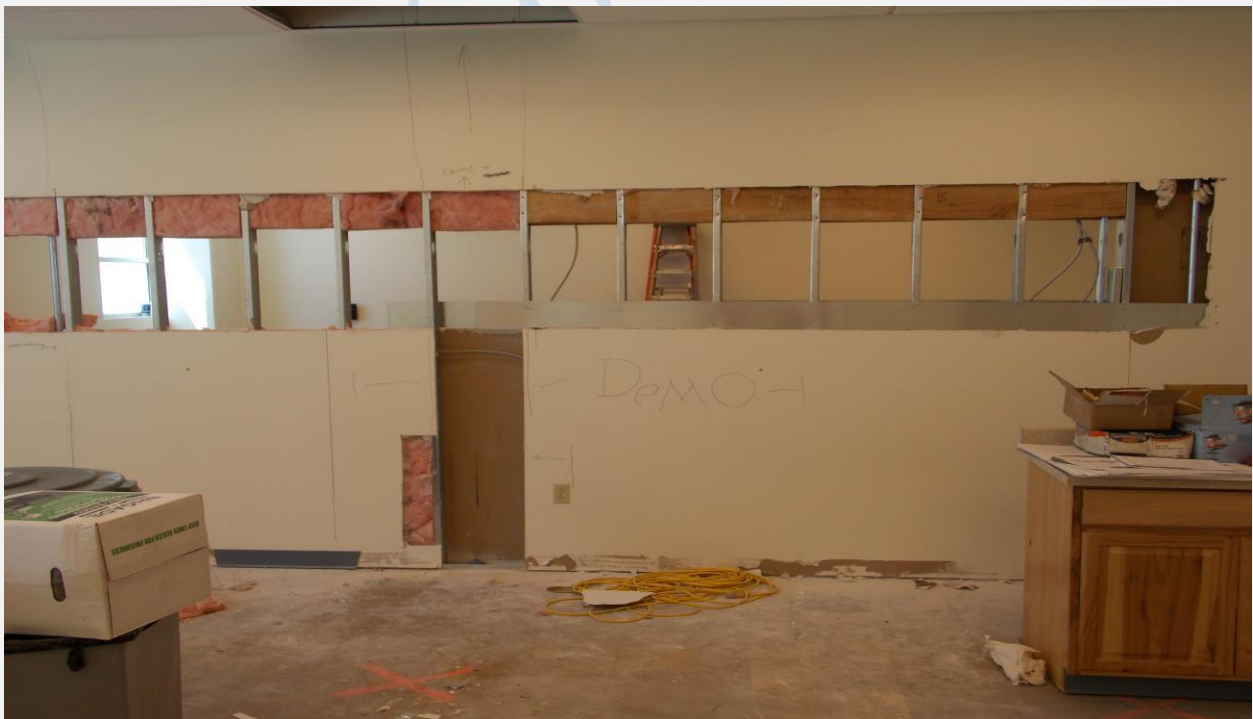
Building 2 Second Floor Demolition for EMS
