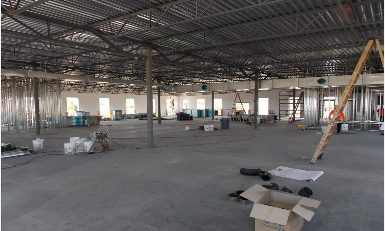
Second Floor Window Installation/Weather Proofing and Framing for Drywall
