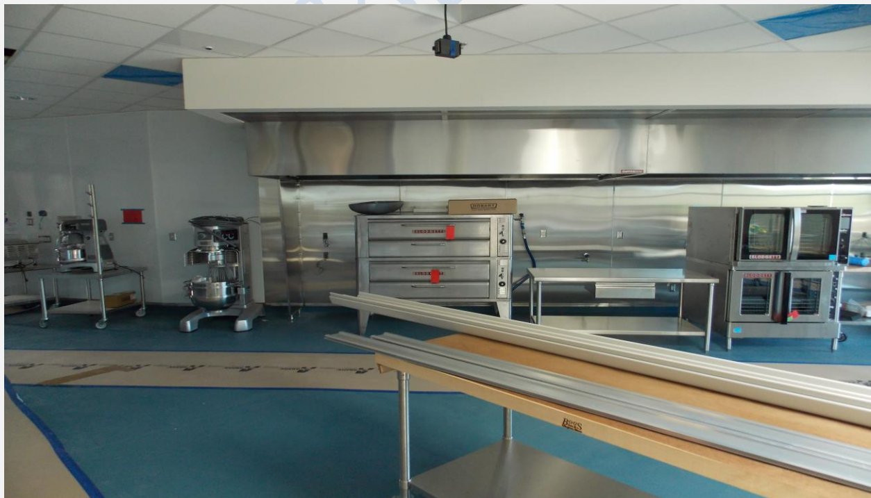
Setting Equipment in Pastry Kitchen
