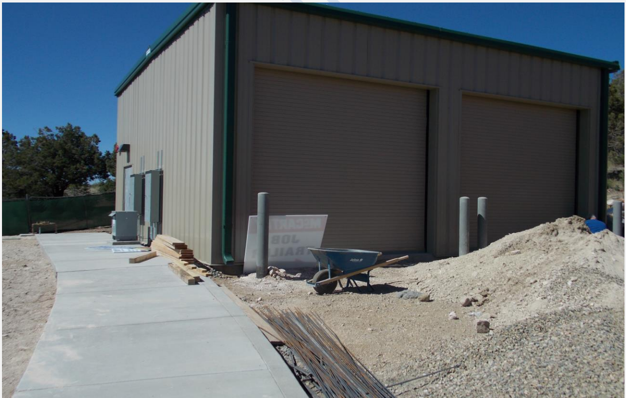
New Sidewalk at EMS Garage
