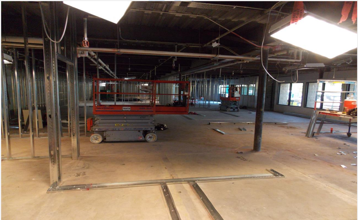
Building 15 First Floor Framing
