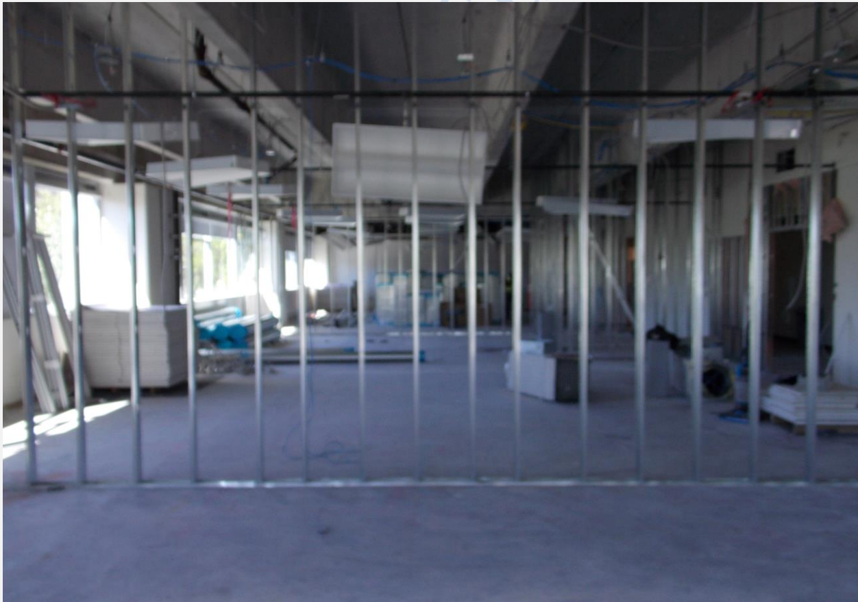
Building 1 Second Floor Framing for Visual Arts Programs
