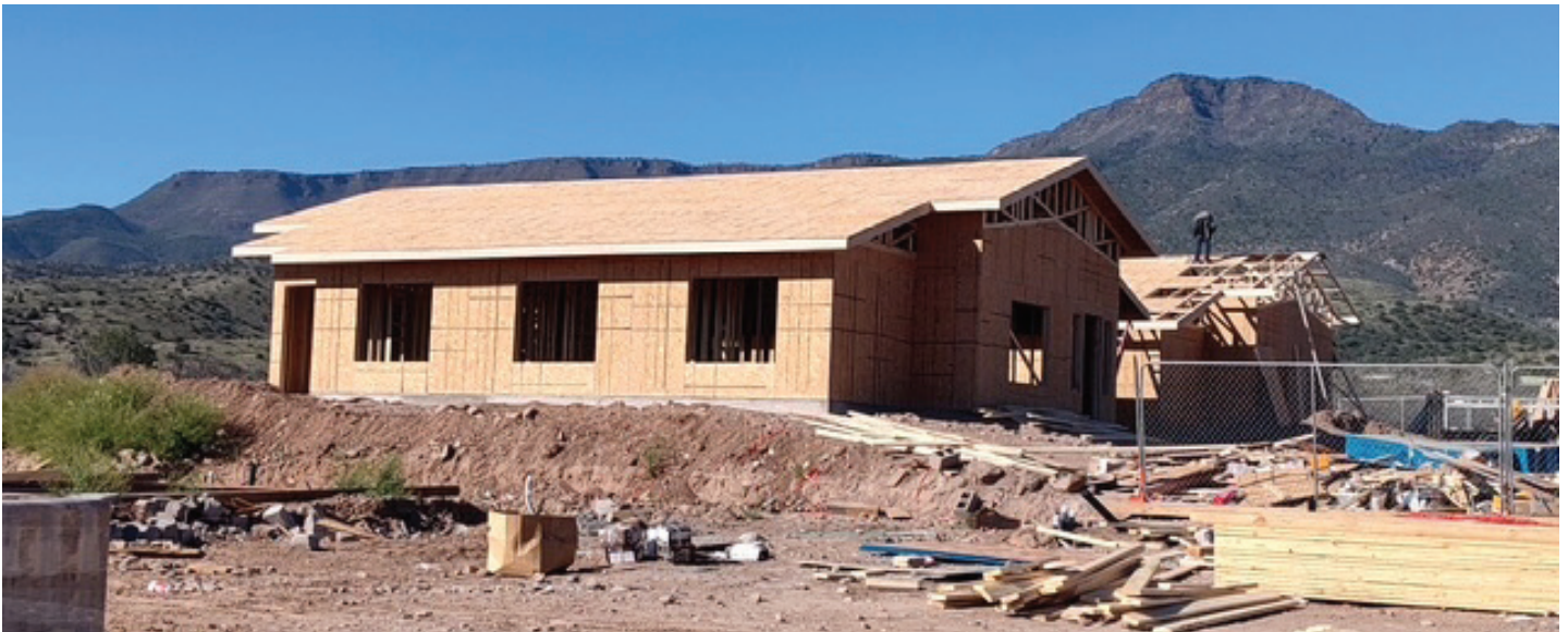
Housing in progress on the Verde Valley Campus.
