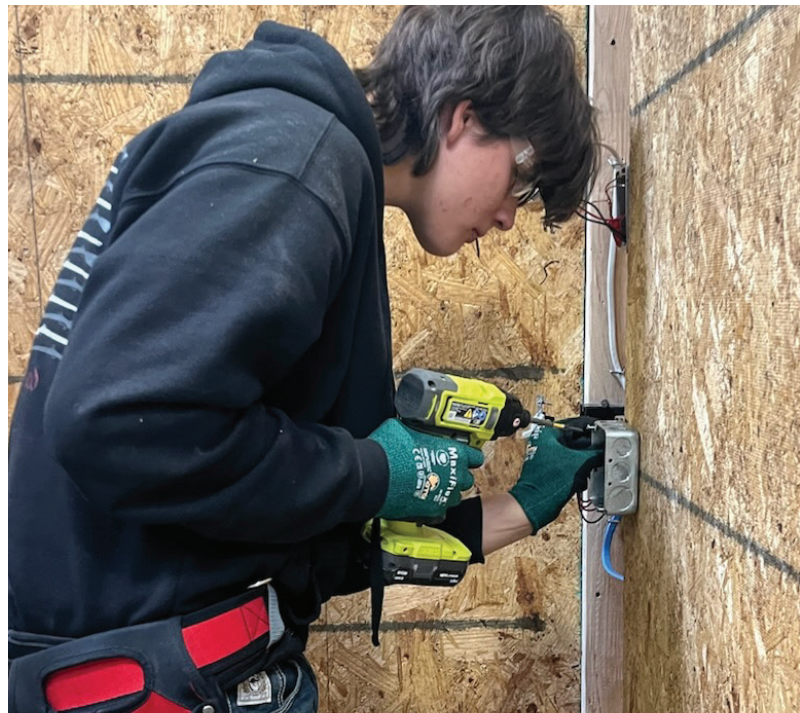
Electrician student making progress for Verde Valley Campus housing.
