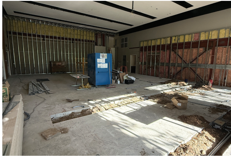
Community Room, 19-147, construction in progress.
