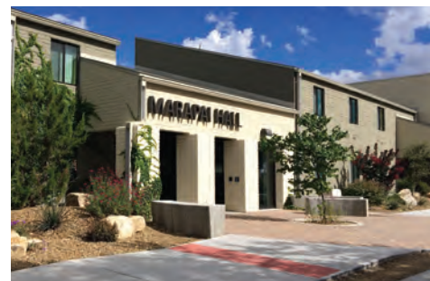
Marapah Residence Hall on the Prescott Campus.
