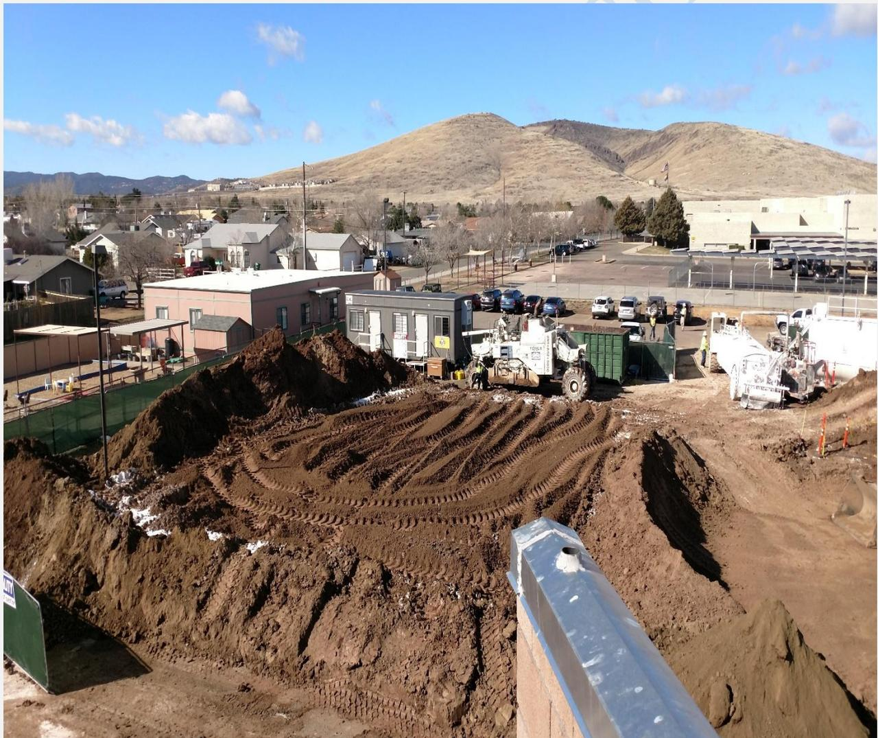
Lime Treatment in Preparation for Foundation Compaction
