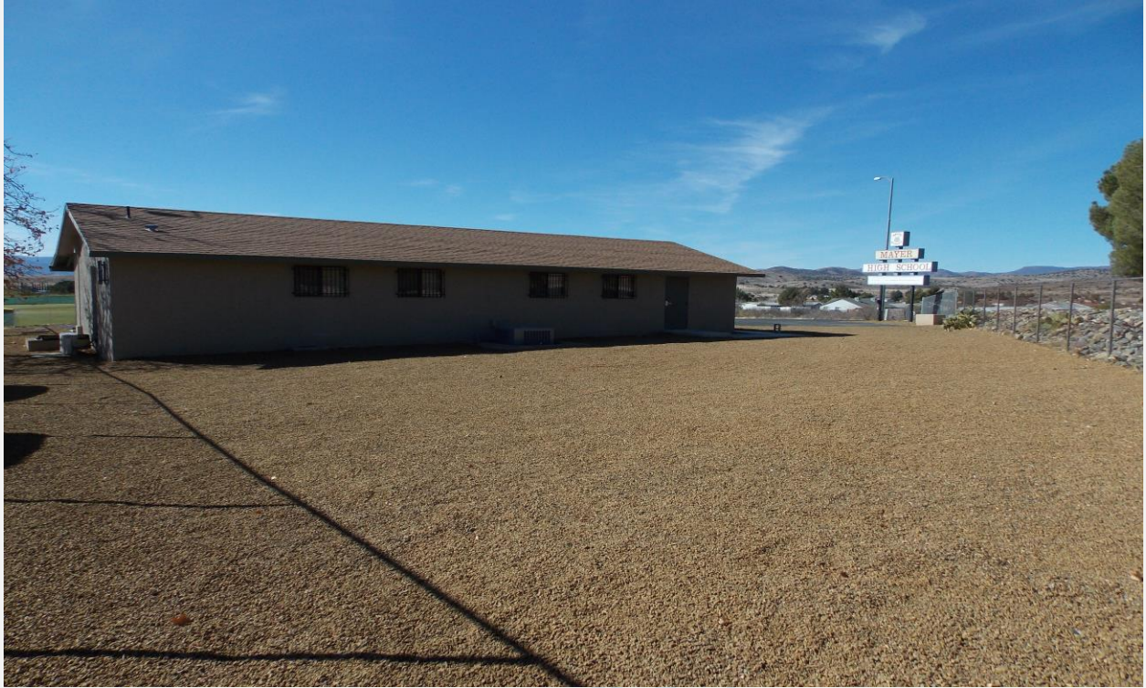
Backside of Building Cleaned up and Ready for the Grand Opening
