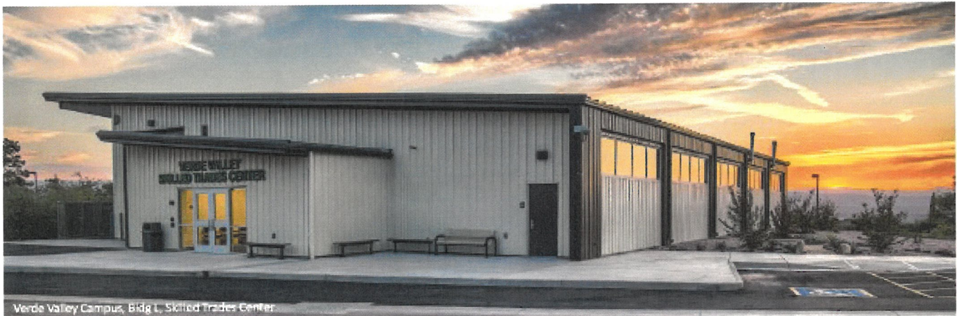
Verde Valley Campus, Bldg L, Skilled Trades Center
