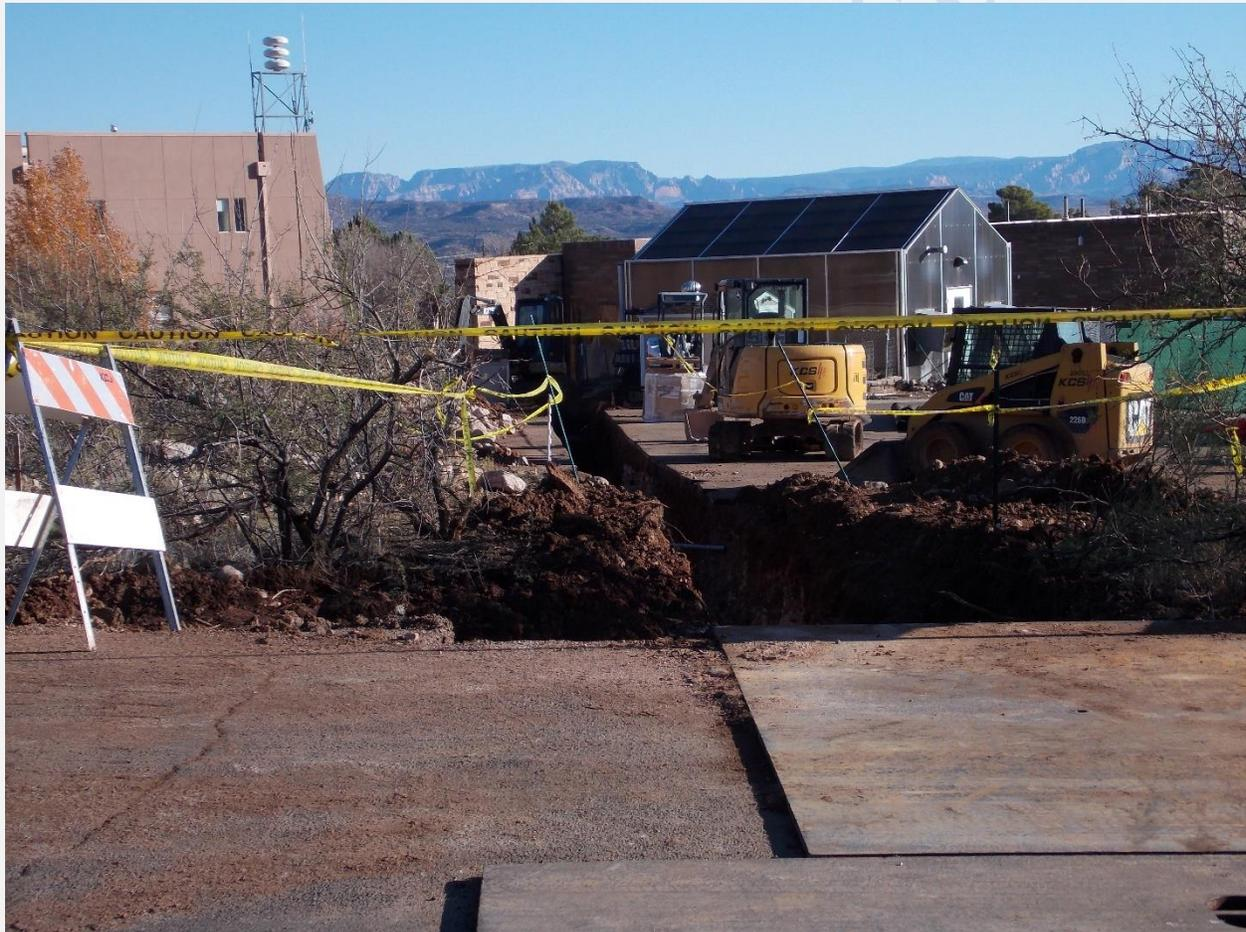
Trenching for Water Line on December 17 for Fire Sprinkler System for Building L
