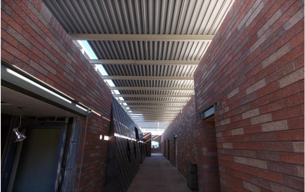
Roof Decking Enclosing Second Floor
