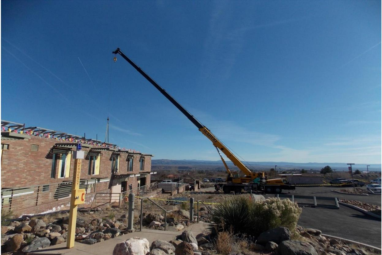
Setting Structural Steel for New Roof
