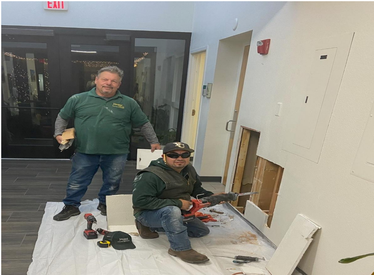
Technician III Plumber, Mike Murphy, and Technician III Trades, Jaime Hernandez, installing a bottle filling station in building 32
