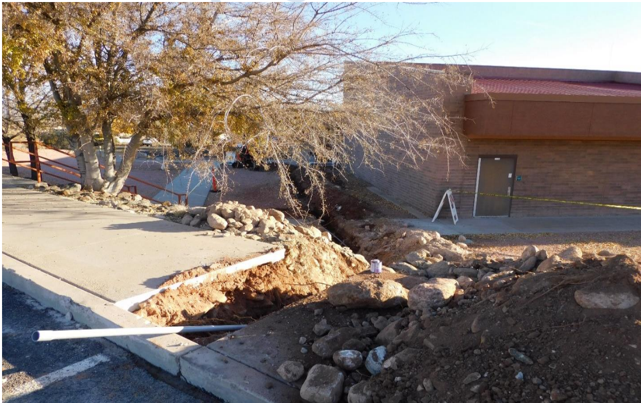
EV Charging Station utility installation near building I
