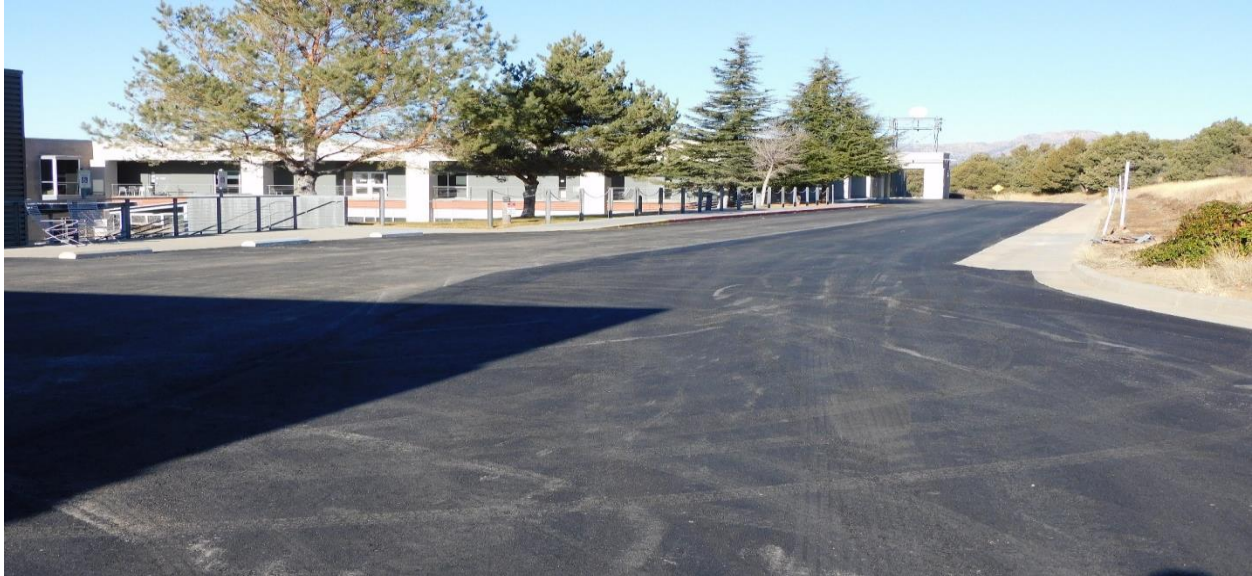
Roadway behind buildings 3 and 4
