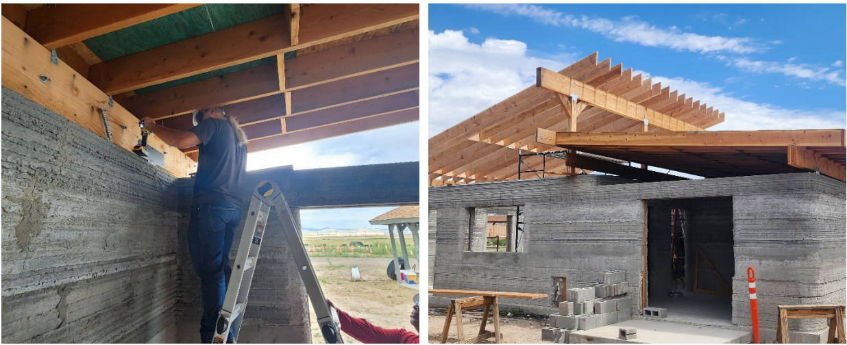
Construction student working on 3D Concrete Printed House
