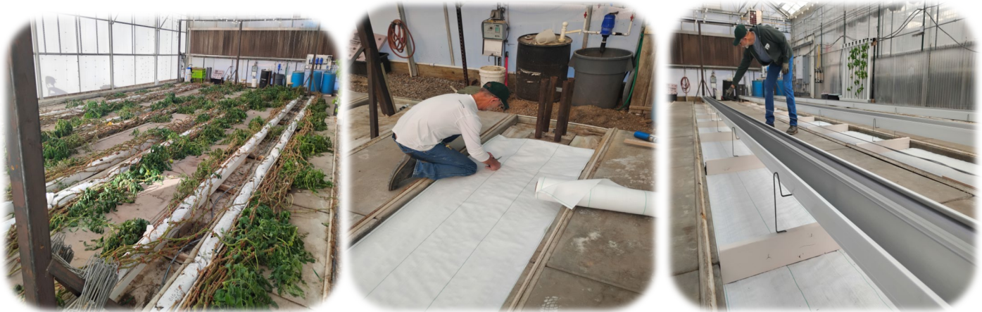
New gutters and irrigation upgrades at YC's hydroponic tomato operation
